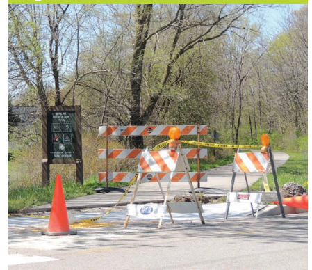
Installation of an ADA compliant crossing at the intersection of Bug Line Trail and Christman Road
