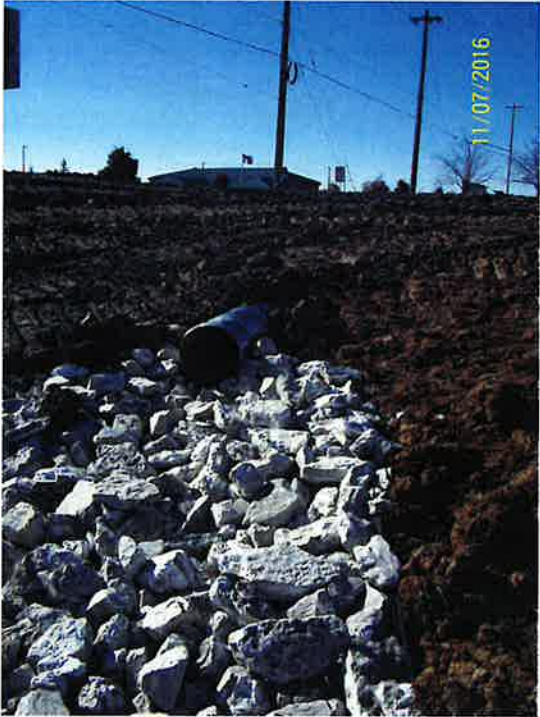
Storm Water Outlet ST010926
