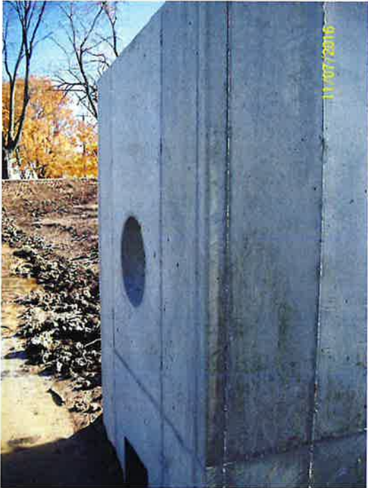
Storm Water Overflow Structure ST014911
