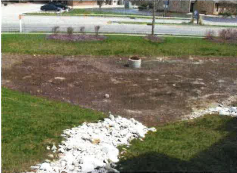
Pond I.D. #SWP4N008 Looking northeast across basin.
