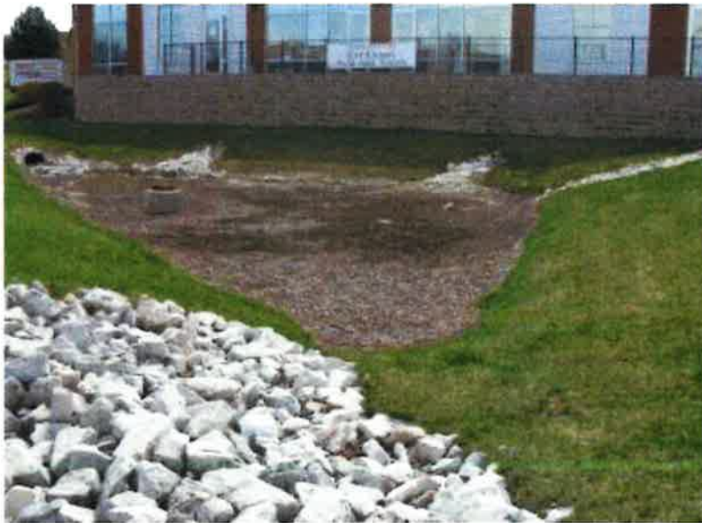
Pond I.D. #SWP4N008 Looking south across basin
