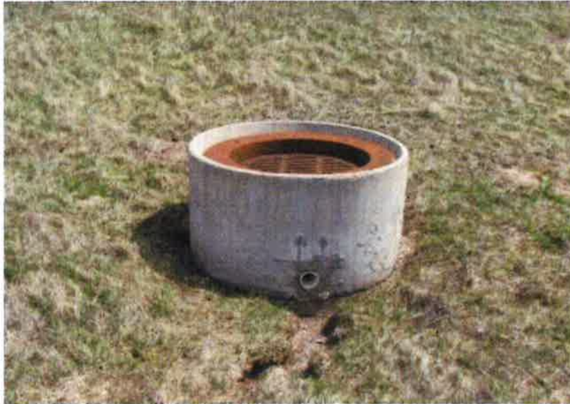
Pond I.D. #SWP02s001 Outlet structure
