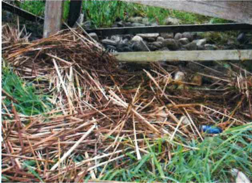
Pond I.D. #SWP02s002 Basin spillway—south side of basin
