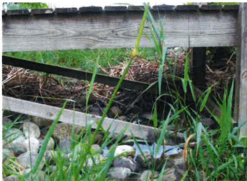
Pond I.D. #SWP02s002 Basin spillway on south side of basin
