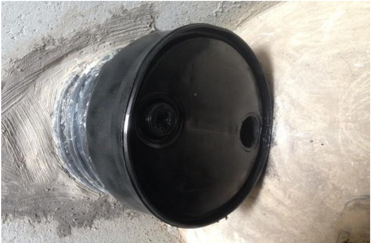
Menomonee Falls Assisted Living –Manhole at discharge of underground storage, orifice restricting flow.
