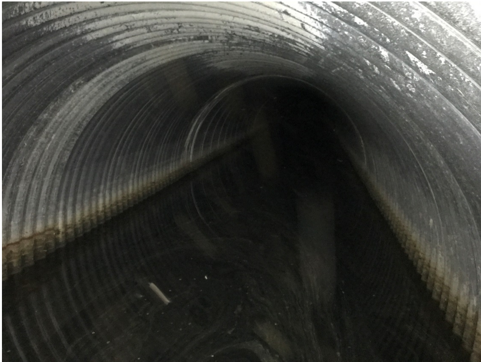
Underground System North Chamber - Looking West
