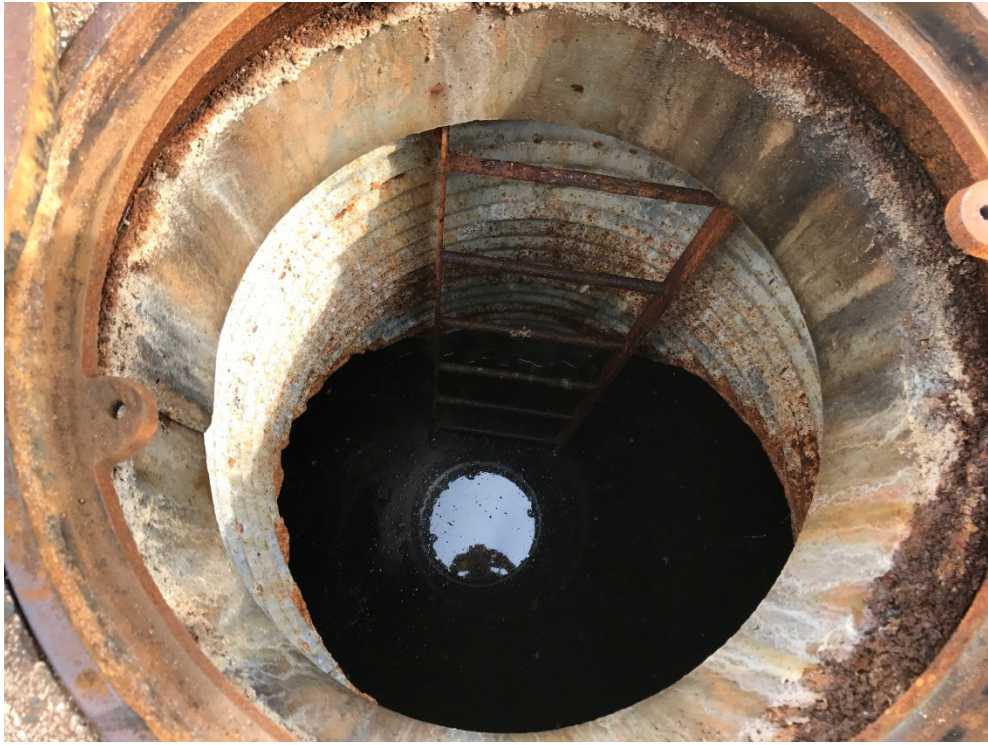
Underground System North Chamber Access Manhole - Looking North
