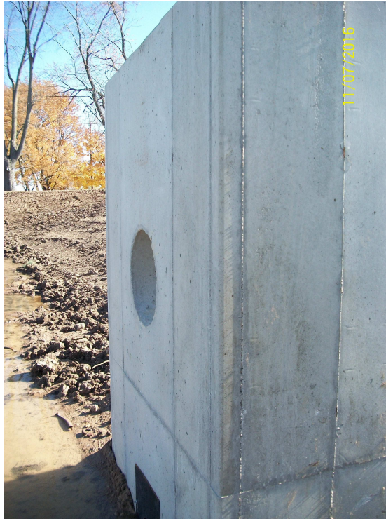
Storm Water Overflow Structure ST014911
