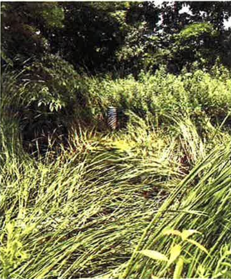
Photo showing cattails at bottom of pond and riser structure
