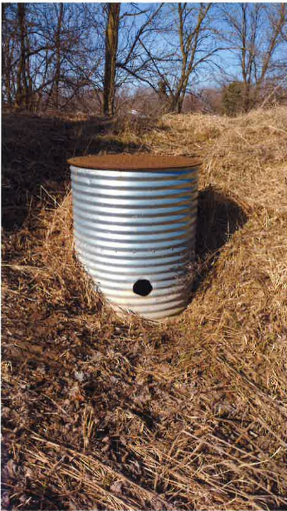
Pond SWP3N001 – 42" CMP Outlet Structure
