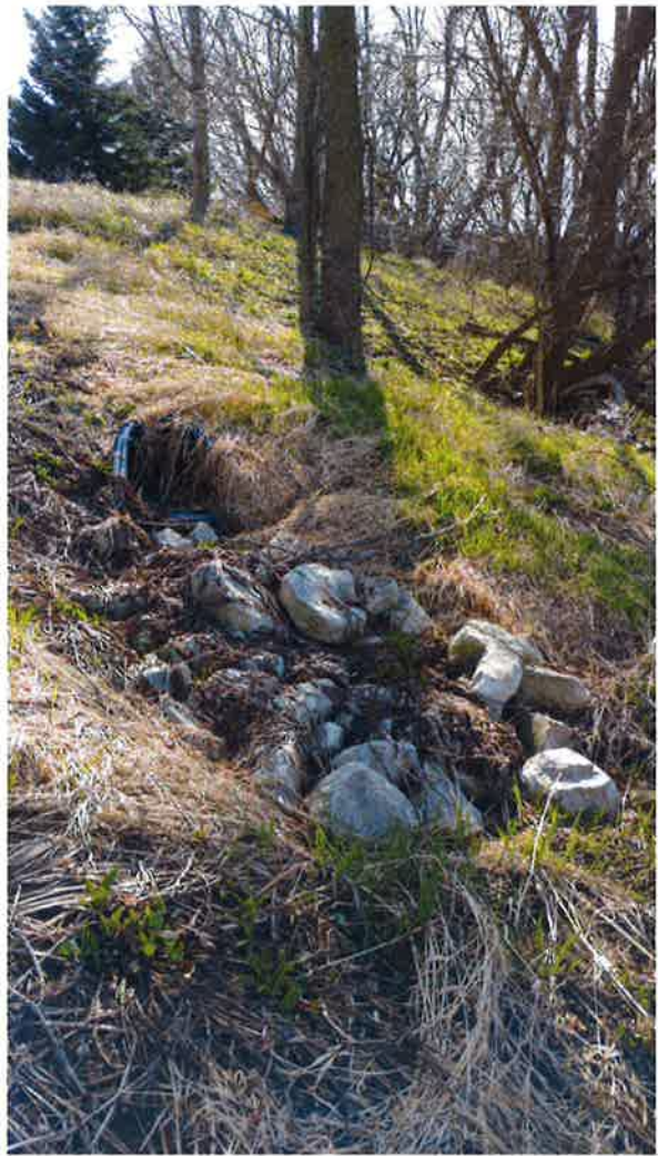
Pond SWP3N001 – 12" Outlet Discharge End
