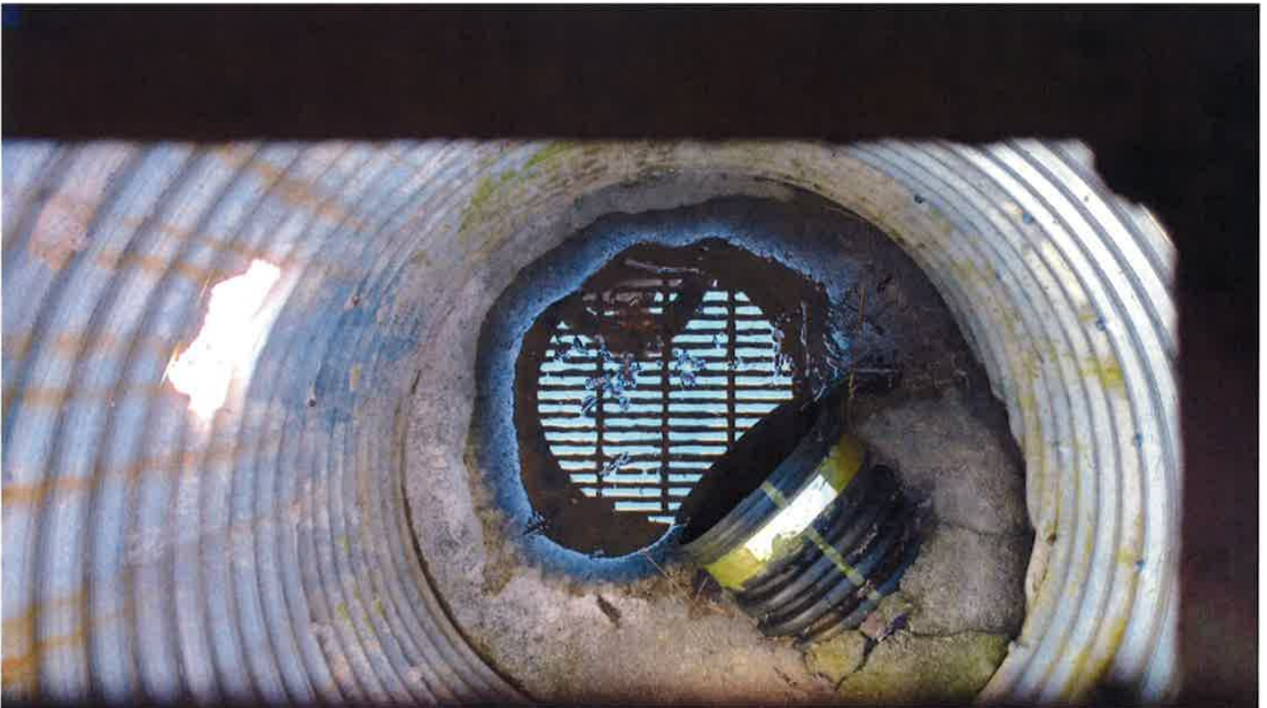
Pond SWP3N001 – Looking inside 42" CMP Outlet Structure
