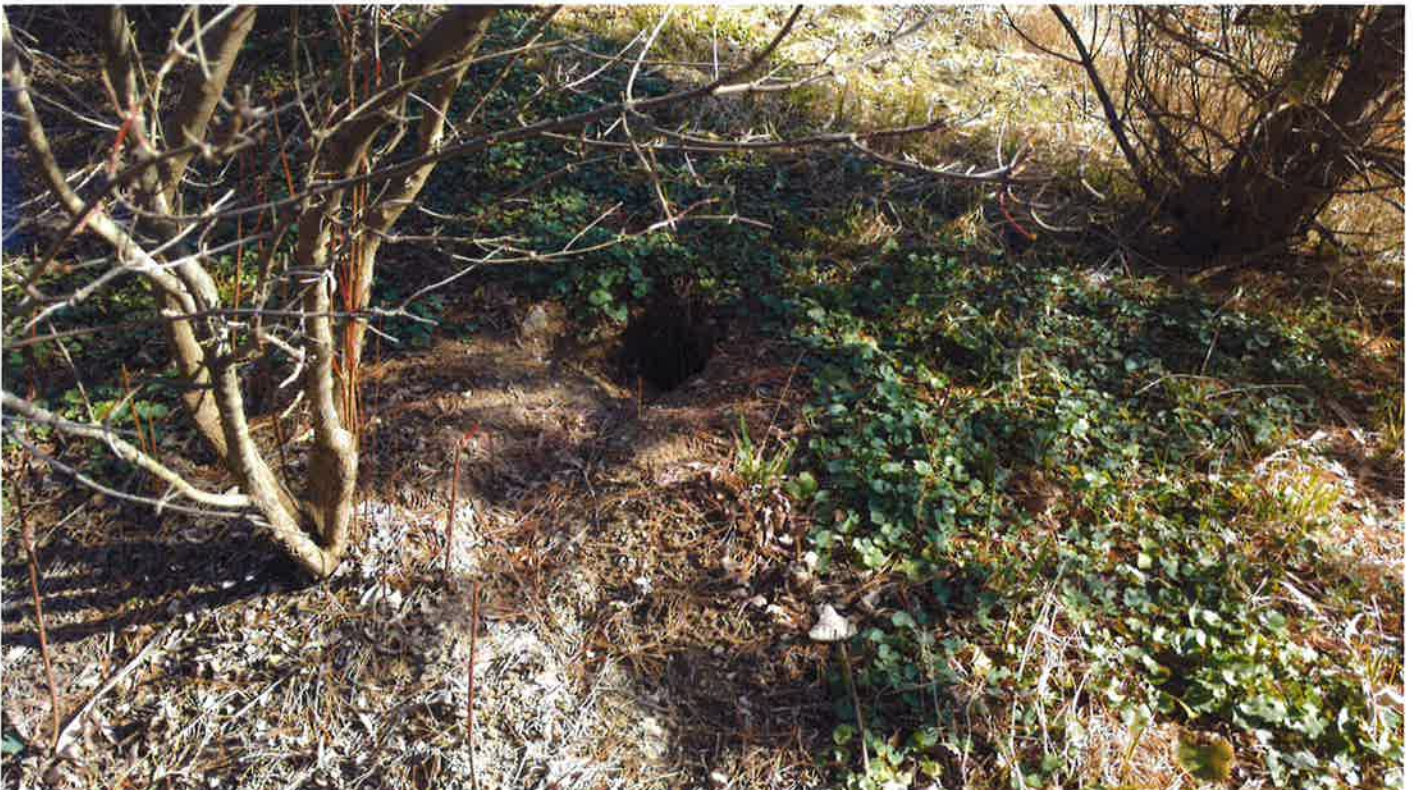
Pond SWP3N001 – Rodent burrow along the Northern berm west of the Emergency Spillway
