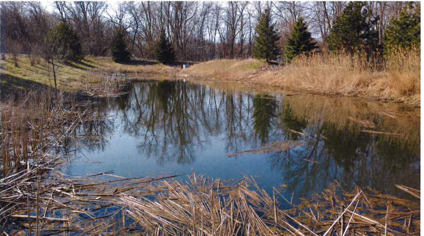
Pond SWP3N001 – Looking Southwest towards Outlet Structure
