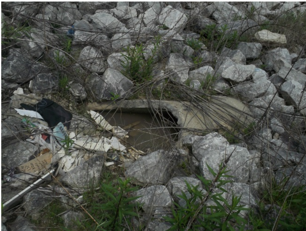
Figure 4: North 24" RCP (Outfall the debris)
