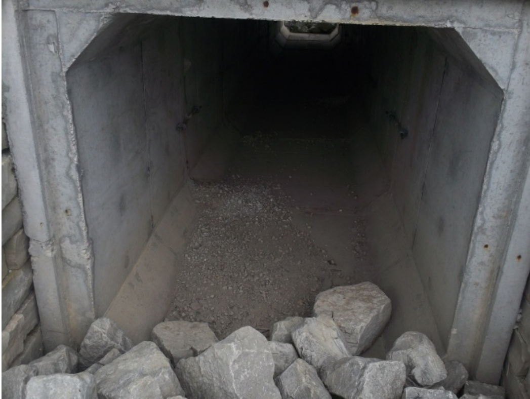
Figure 5- Equalization Pipe between SWP13S007 and SWP13S005
