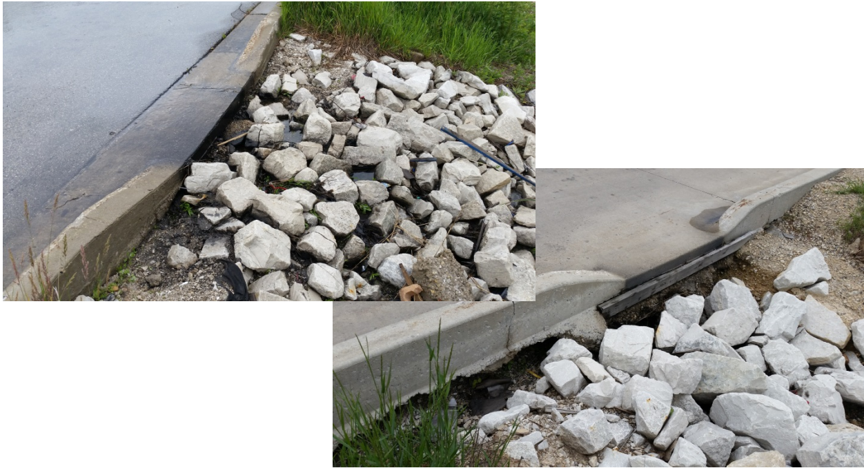
Photos 8 & 9: Flows carried downslope toward basin from curb cuts at Quad Graphics plant has led to some undermining of hard surface pavement.
