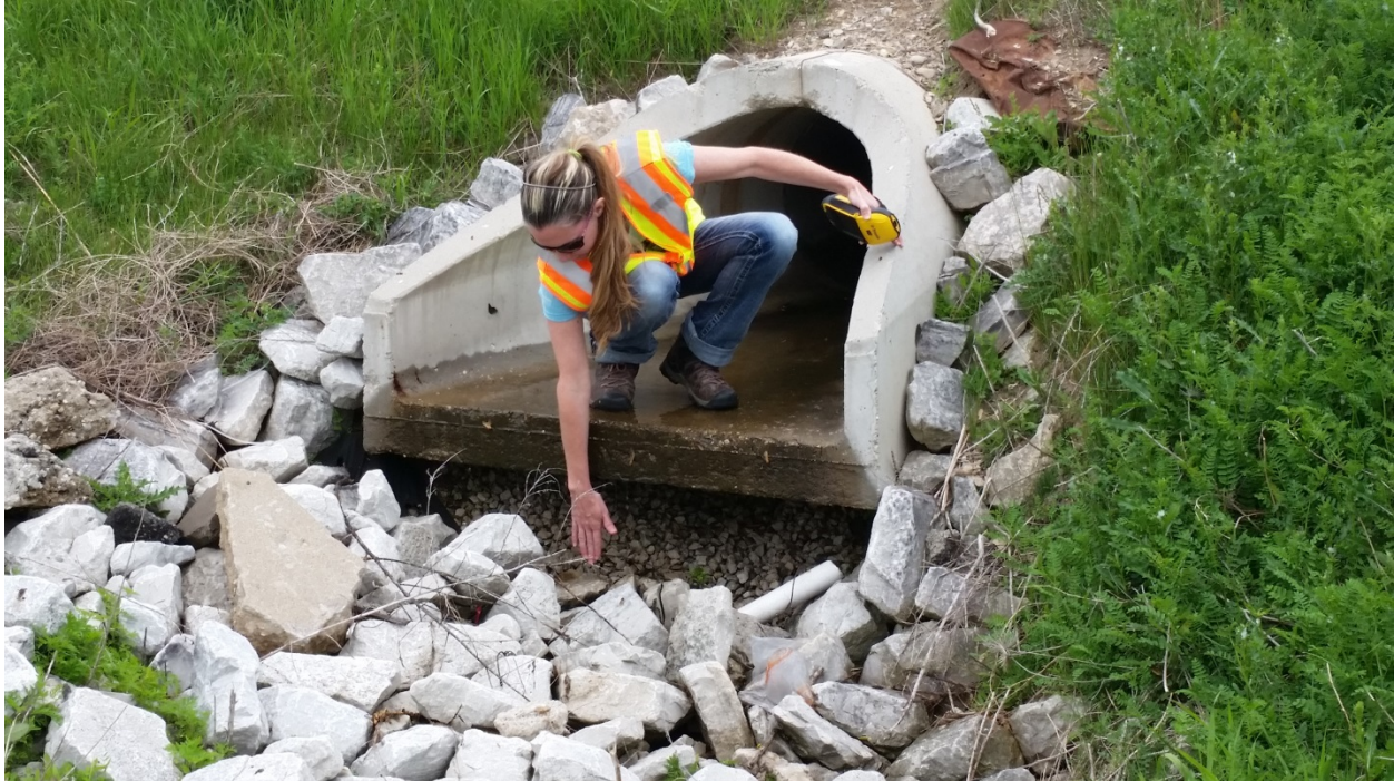
Photo 10: Rip rap has moved as a result of flows and gravity. Rip rap should be replaced to minimize voids between flow paths and structures. *NOTE: In the event that land disturbance will occur as part of basin maintenance, please contact the Village to determine if an erosion control permit or any other permits will be needed.
