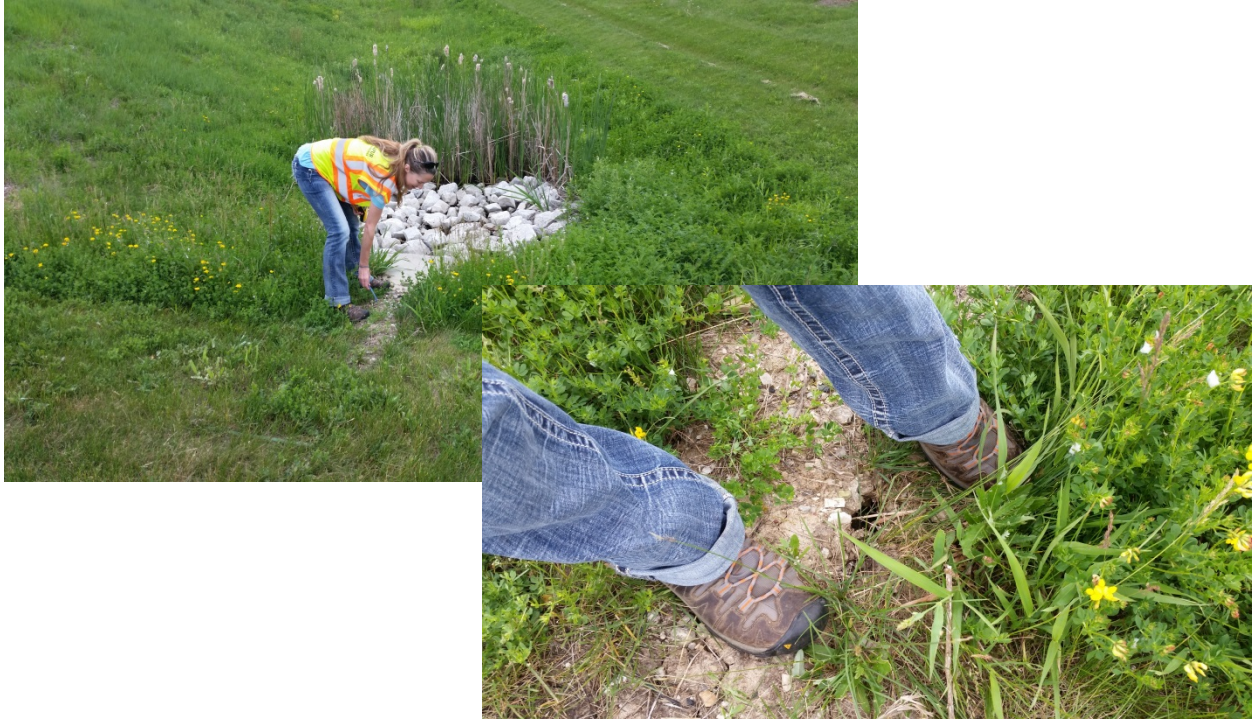
Photos 5 & 6: Top of west pond inlet pipe requires some restoration (replacement of topsoil, seed and stabilization).
