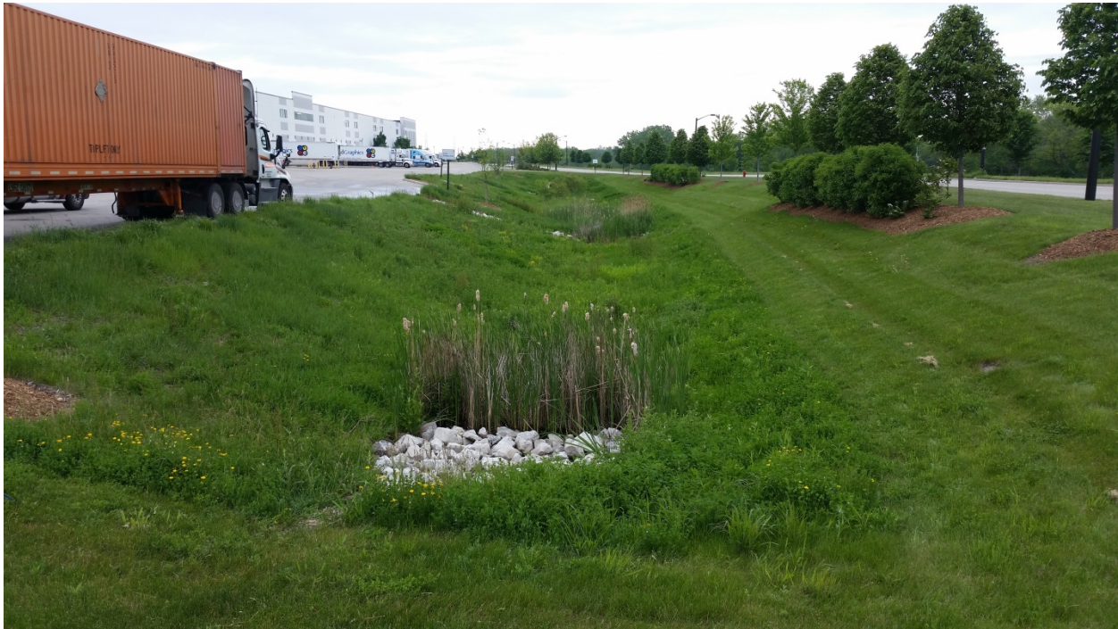
Photo 1: Vegetation along basin banks generally provides adequate cover. Photo taken from west side of basin looking east.
