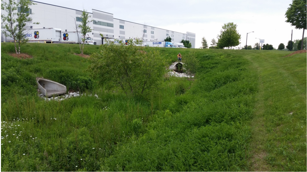
Photo 3: Photo taken looking northeast at pond basin and structures. Woody vegetation (willows) within basin can be removed.
