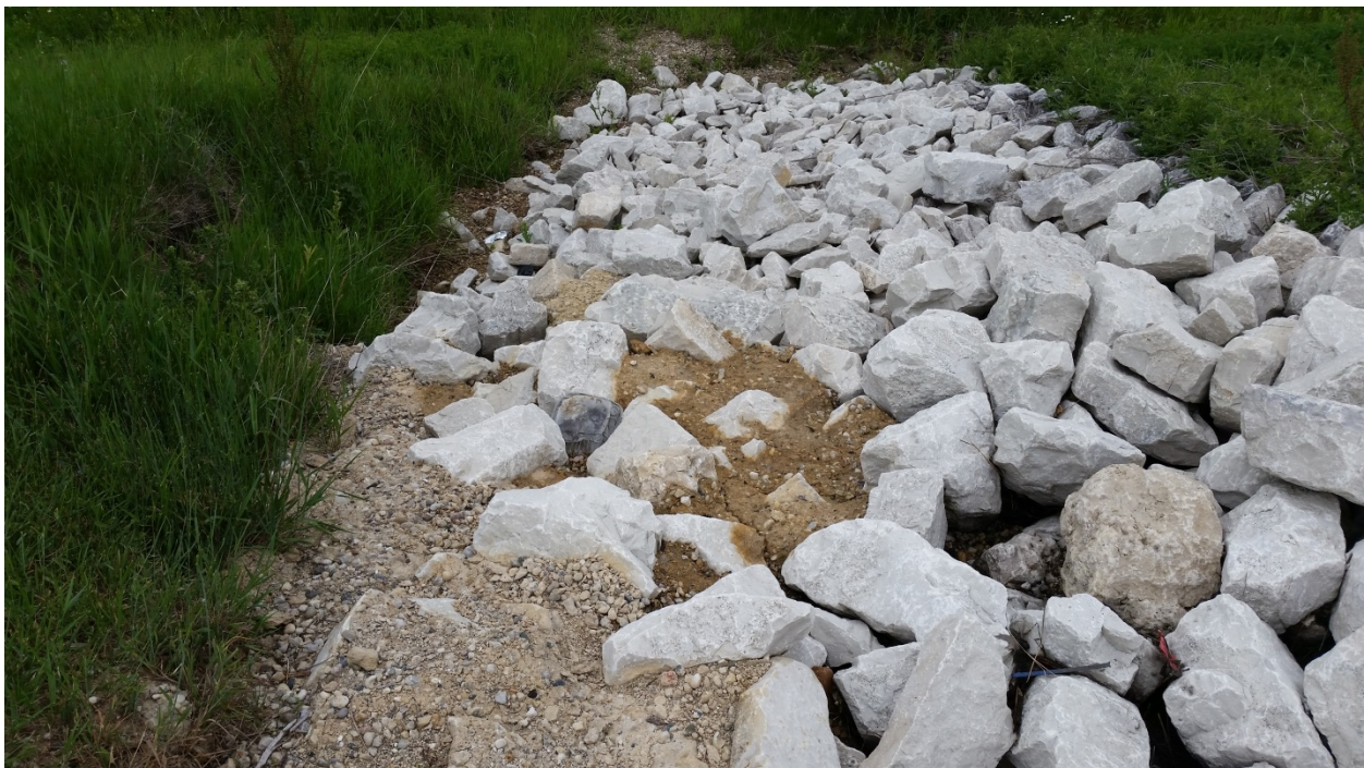
Photo 7: Deposition of sediment within basin. *NOTE: If removal of sediment within basin is planned, make sure to contact local (Village of Menomonee Falls) and State (Department of Natural Resources) regulators for any prior authorization/permitting which may be necessary. Sediment may need to be tested prior to transport to ensure proper precautions are taken for disposal.
