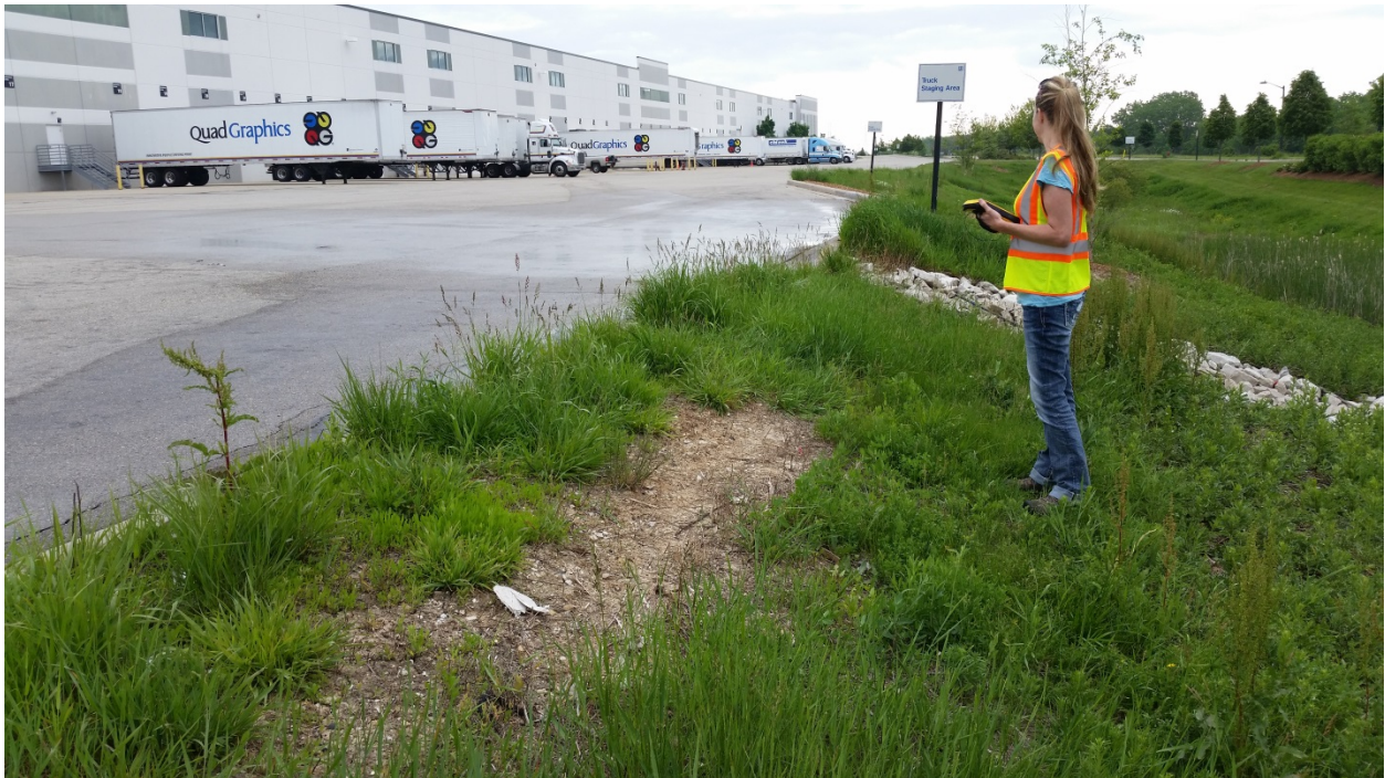
Photo 4: Flows carried downslope toward basin have led to some scouring particularly on north side of basin. Some additional seeding and restoration may be necessary as well as potentially replacing topsoil. *NOTE: In the event that land disturbance will occur as part of pond maintenance, please contact the Village to determine if an erosion control permit or any other permits will be needed.
