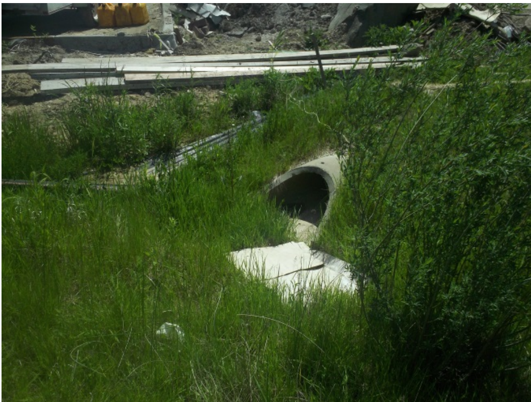
Figure 2: 15" Reinforced Concrete Outfall Located on the Southeast Portion of Pond
