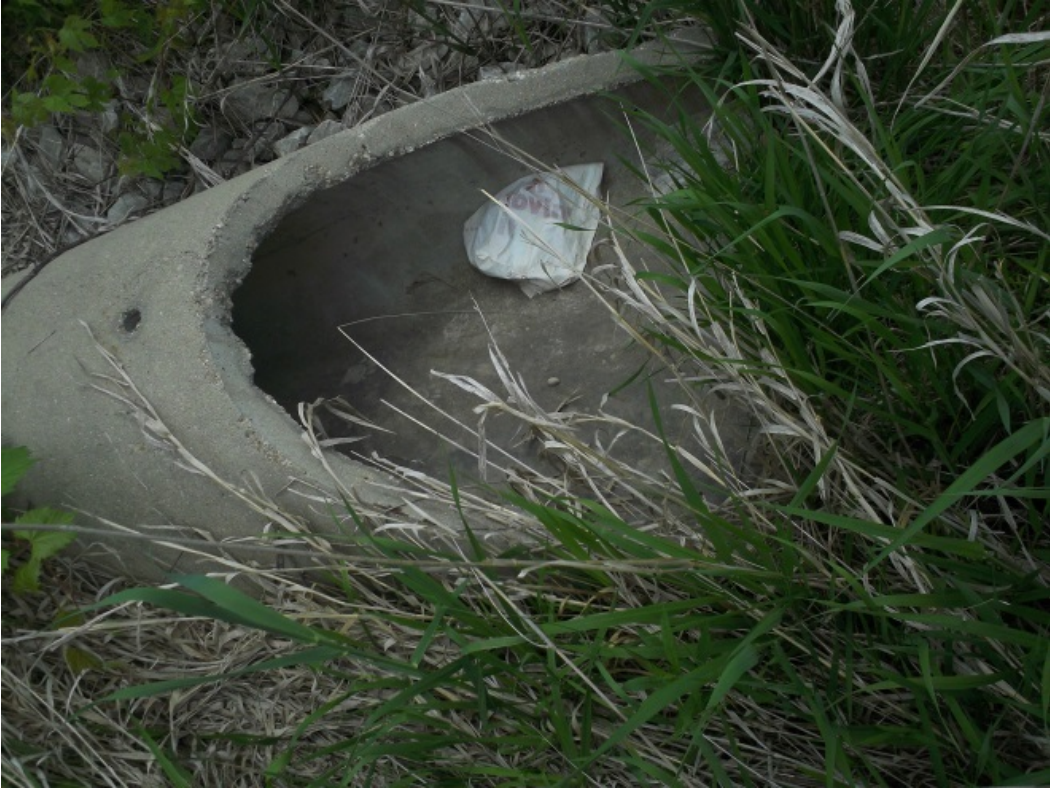
Figure 2- View of the 24" RCP Outlet Structure
