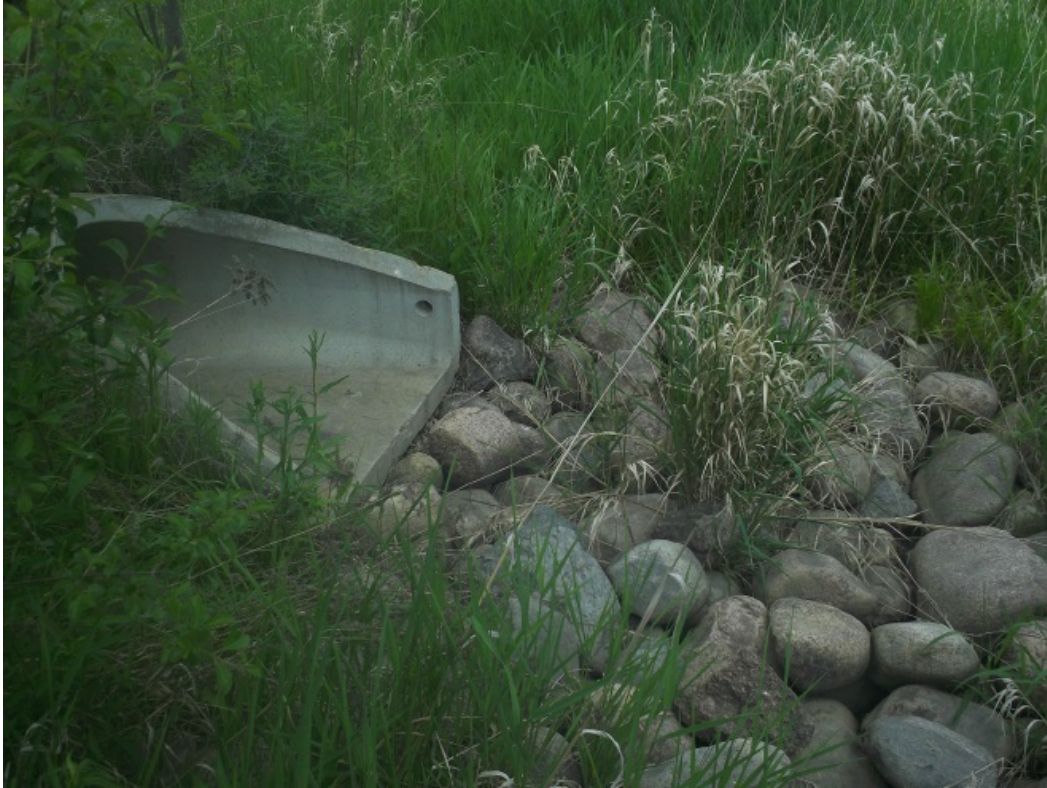
Figure 3- View of 15" RCP Outfall Located on the North End of Pond
