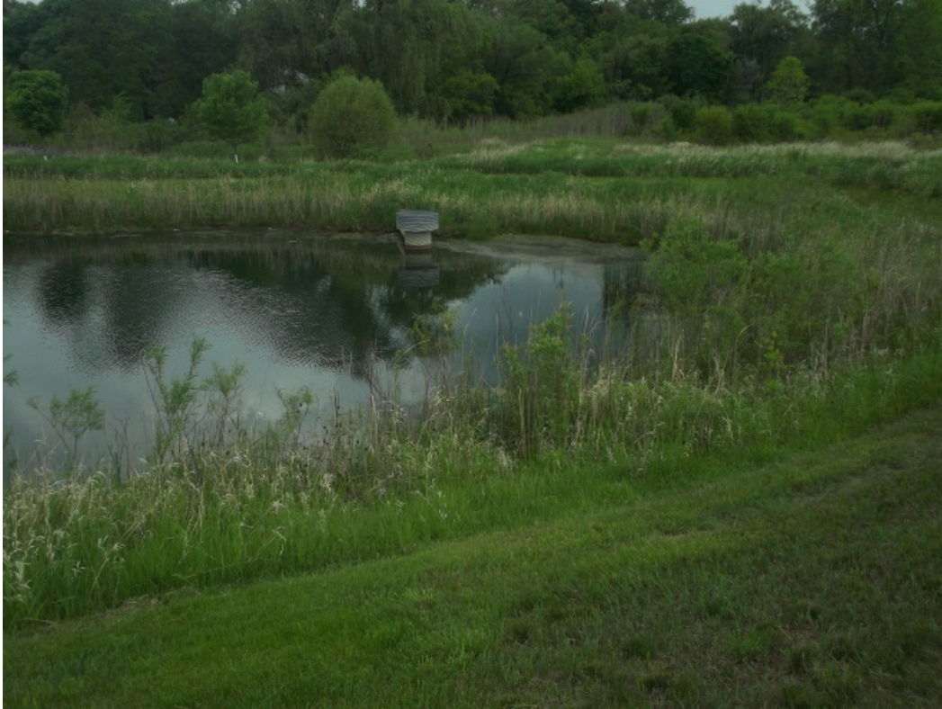
Figure 3: Outlet Structure Located on the North end of Pond
