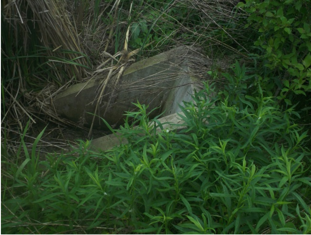
Figure 3: Overview of Outlet Structure
