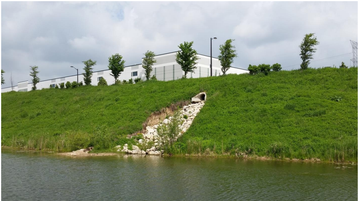
Photo 6: Flows carried downslope toward pond have led to some scouring along pond bank. Some additional rip rap underlain with geotextile fabric may be needed in areas where scour around existing rip rap has occurred. *NOTE: In the event that land disturbance will occur as part of pond maintenance, please contact the Village to determine if an erosion control permit or any other permits will be needed.
