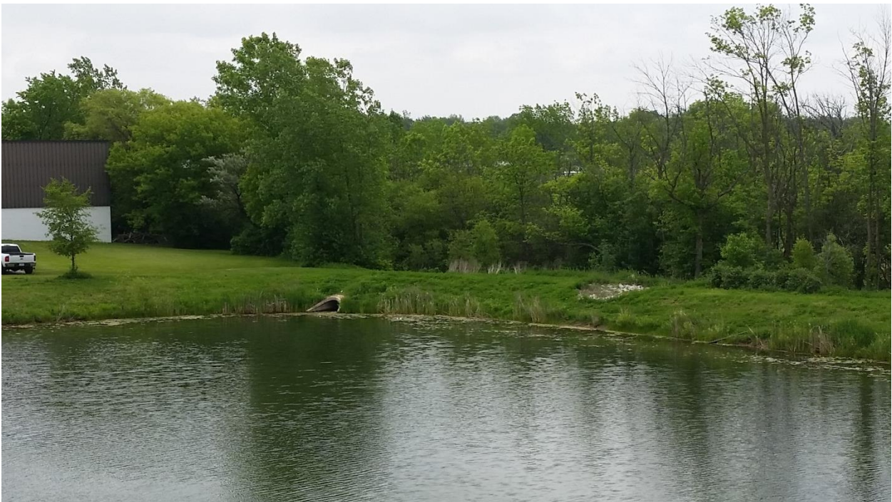
Photo 8: Noted no obstructions at outlet control structure or at emergency overflow spillway during inspection.
