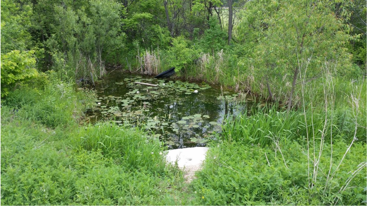
Photo 7: Stormwater pond outlet structure located on southeast end of pond. Outlet is in fine condition, noted no obstructions in outlet. Downstream of outlet is silt fence which had likely been placed with original development. It should be removed so it doesn't cause an obstruction.
