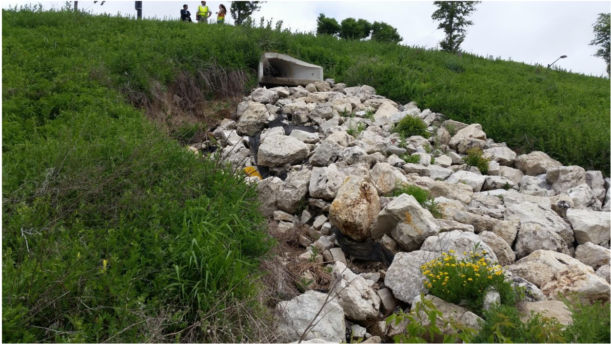
Photo 3: Erosion at northern pond inlet.
