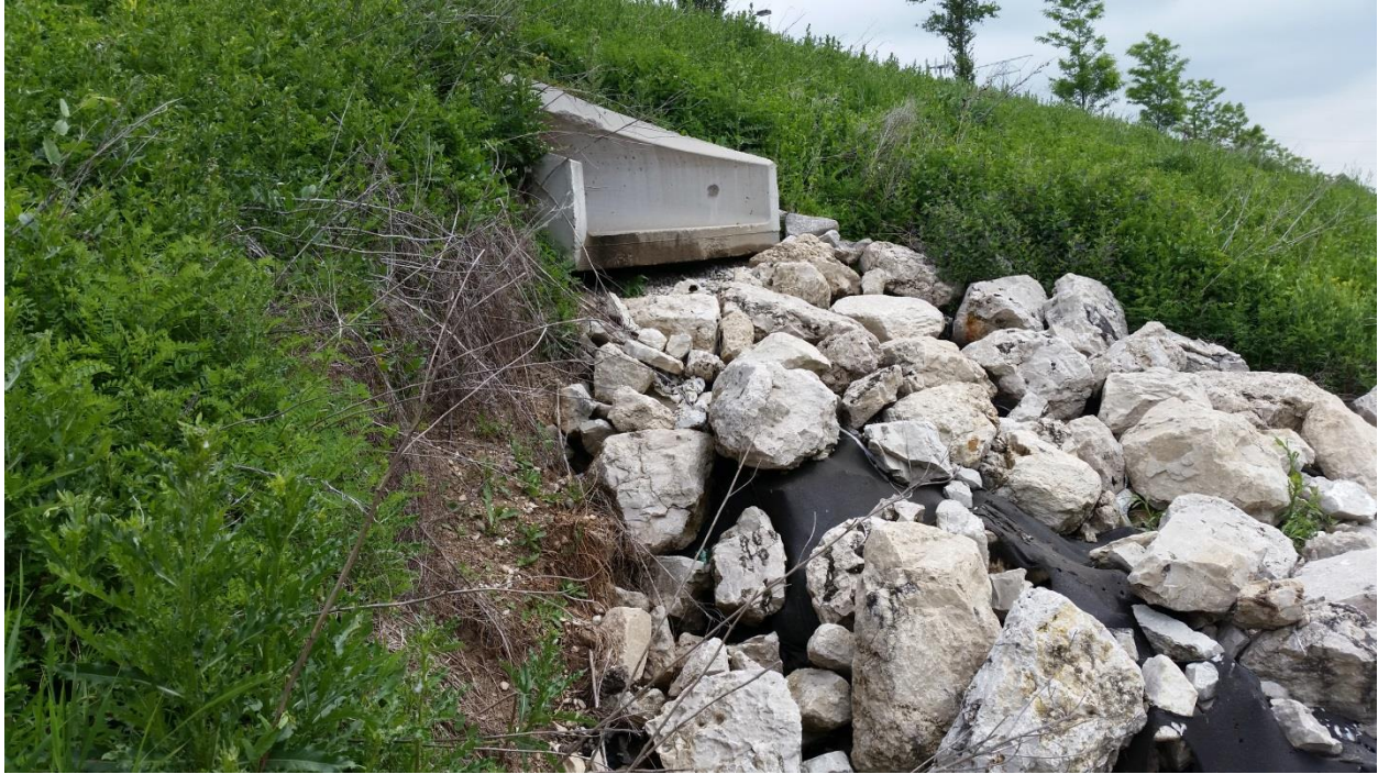
Photo 5: At pond inlets rip rap has become displaced, leaving geotextile fabric beneath exposed.
