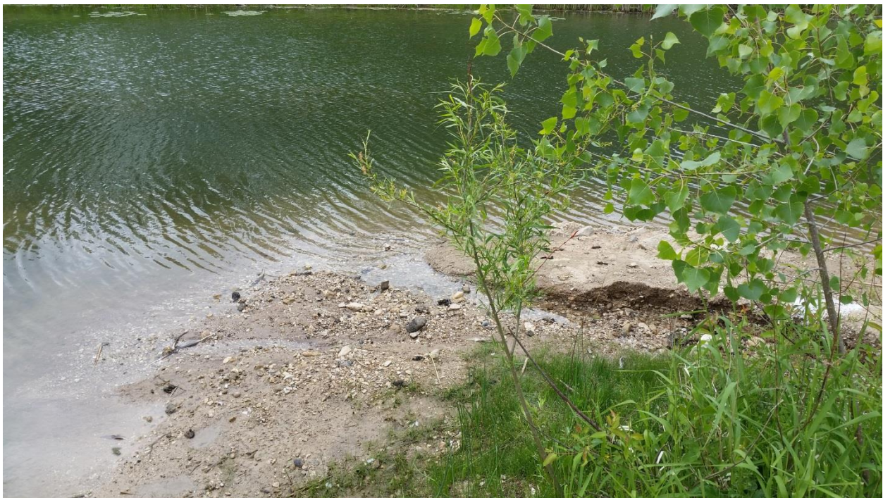
Photo 4: Deposition of sediment within basin of pond. *NOTE: If removal of sediment within pond is planned, make sure to contact local (Village of Menomonee Falls) and State (Department of Natural Resources) regulators for any prior authorization/permitting which may be necessary. Sediment may need to be tested prior to transport to ensure proper precautions are taken for disposal.
