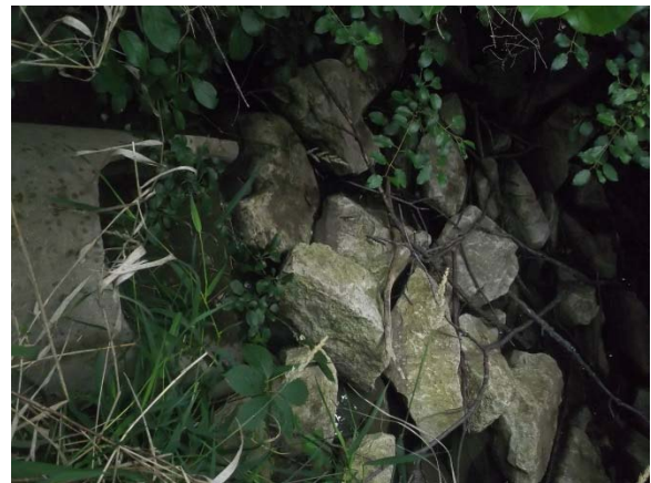
Figure 6: Outfall for the Pond Structure, Located Southeast of the Pond
