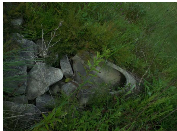
Figure 5: Overview of Outfall Located on the North Portion of the Pond
