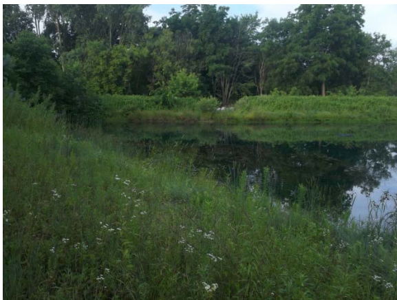
Figure 3: Overview of the Emergency Spillway, Looking East
