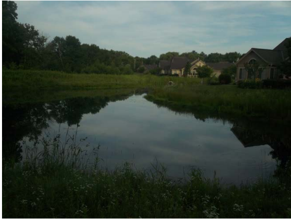
Figure 2: Overview of Pond, Looking West
