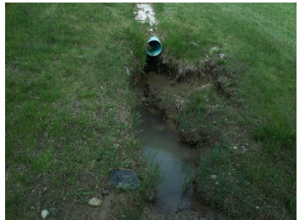
Figure 6: 6" PVC Outfall Located on the West Slope of Pond
