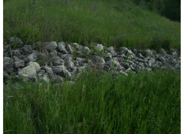
Figure 5: Emergency Spillway Located on the Northeast Portion of Pond
