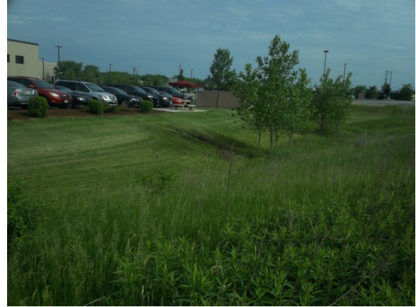
Figure 4: Looking Northwest, Overview of Dry Pond (Note: Two Groupings of Tree Growth)
