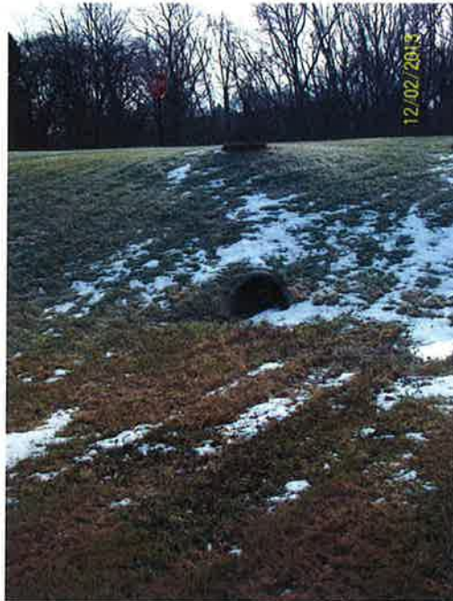
Manhole ST11N026 & Inlet IN11N009
