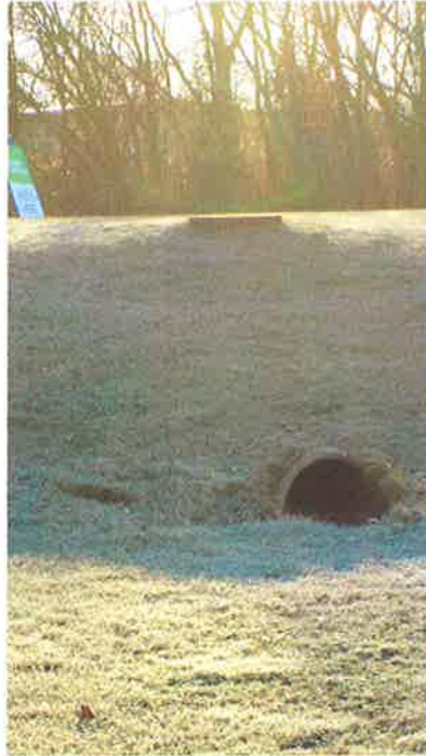
Manhole ST11N026 & Inlet IN11N009
