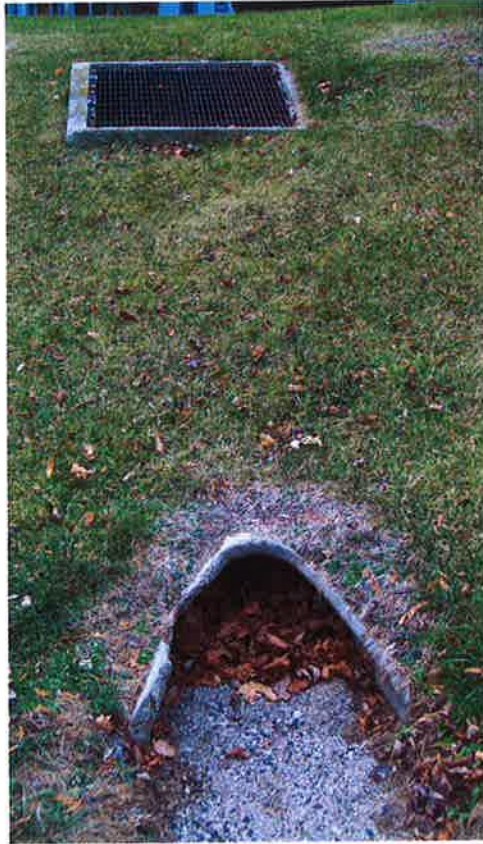
Inlet IN14N003 and Overflow YB14N009
