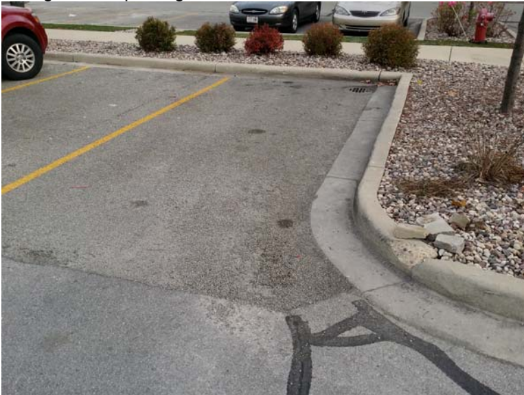
Photo #8: Minor surface spalling is present along the asphalt/concrete joint at numerous locations throughout the parking areas.
