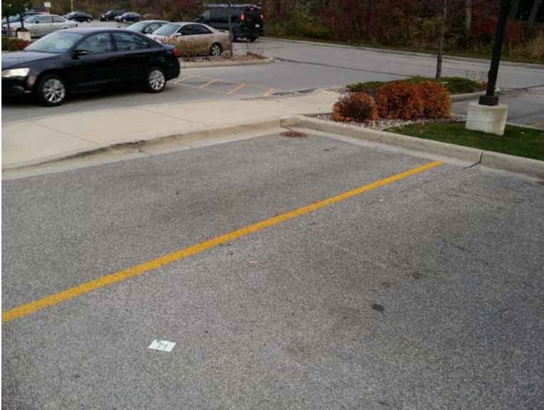
Photo #8: Minor surface spalling is present along the asphalt/concrete joint at numerous locations throughout the parking areas.
