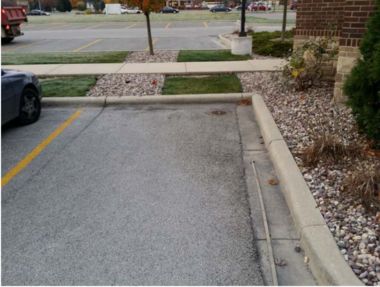
Photo #4: Minor vehicle fluid staining was observed within concrete parking areas.
