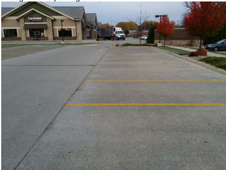
Photo 10: Minor surface spalling is present along the asphalt/concrete joint at numerous locations throughout the parking areas.
