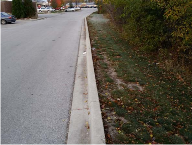
Photo 12: Minor surface spalling is present along the asphalt/concrete joint at numerous locations throughout the parking areas.
