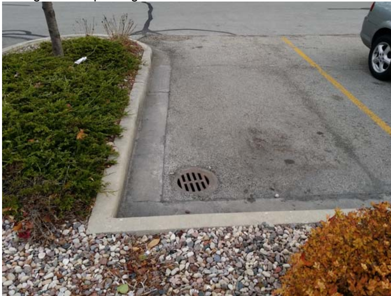
Photo 10: Minor surface spalling is present along the asphalt/concrete joint at numerous locations throughout the parking areas.
