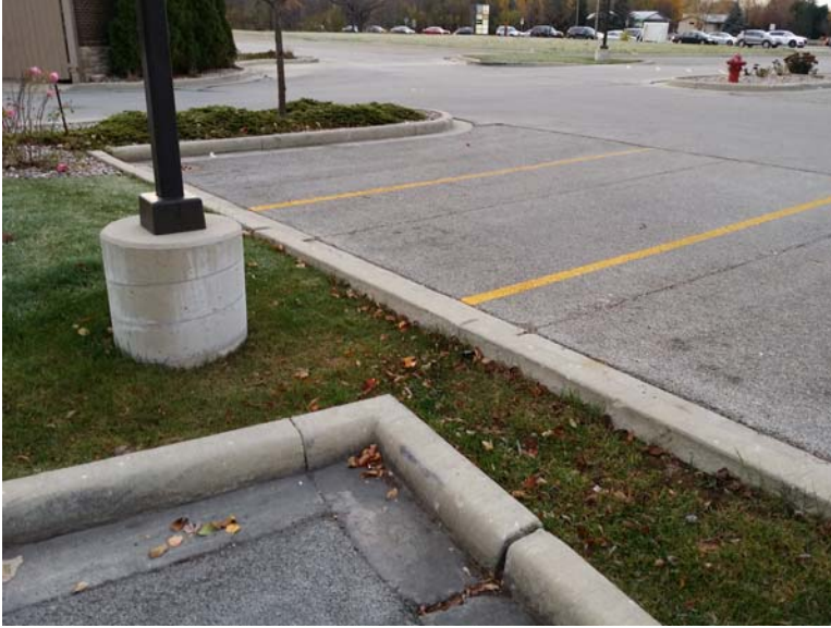
Photo #6: Delivery trucks should be minimized on the porous concrete areas to prolong service life.
