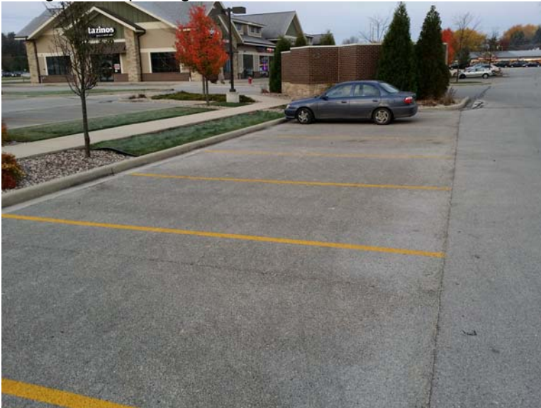
Photo 12: Minor surface spalling is present along the asphalt/concrete joint at numerous locations throughout the parking areas.
