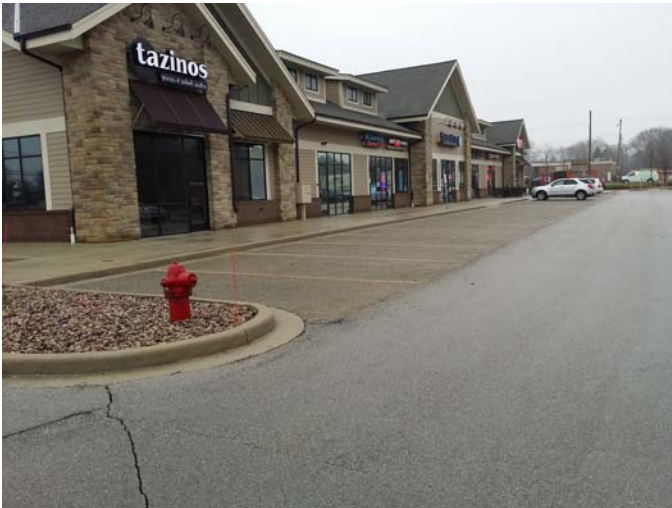
Photo #6: Parking lawn areas showing signs of settlement behind curbs and adjacent to walkways.
