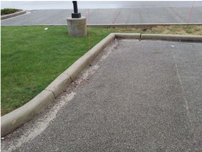
Photo #6: Parking lawn areas showing signs of settlement behind curbs and adjacent to walkways.
