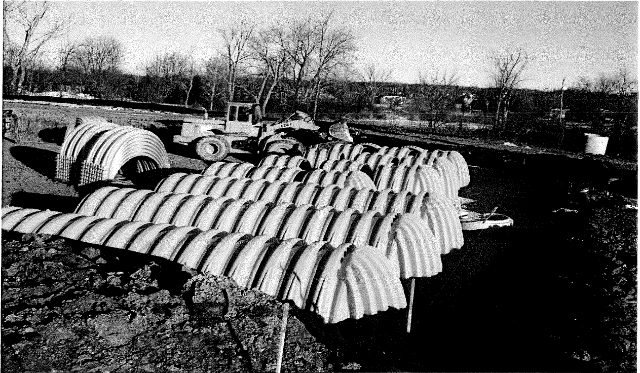
Menomonee Falls Assisted Living- Underground Detention
