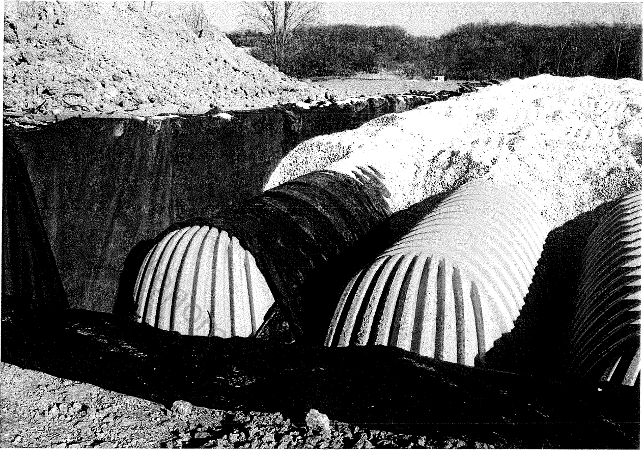
Menomonee Falls Assisted Living- Underground Detention
