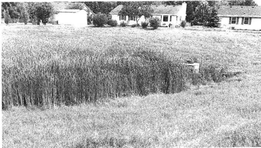
Photo showing cattails at bottom of pond and riser structure.
