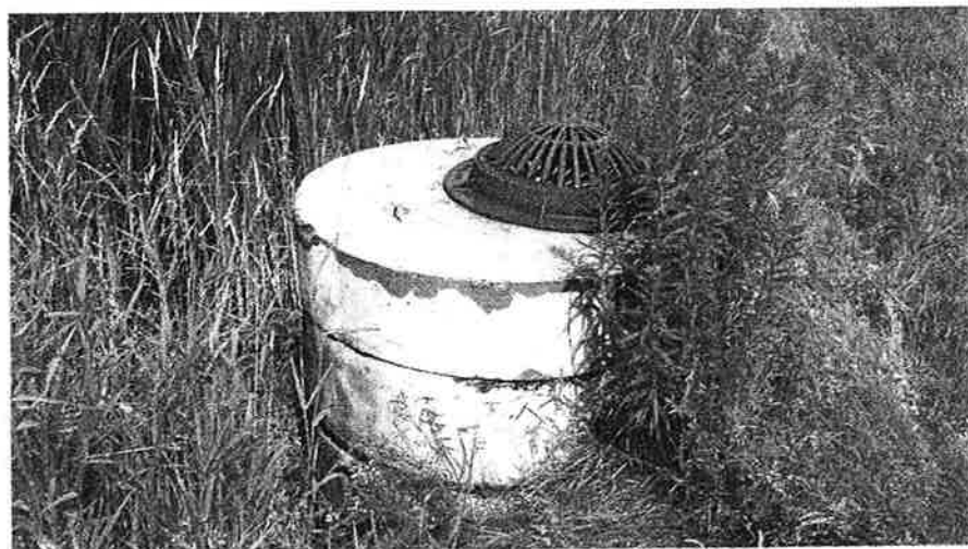
Photo showing riser structure.
