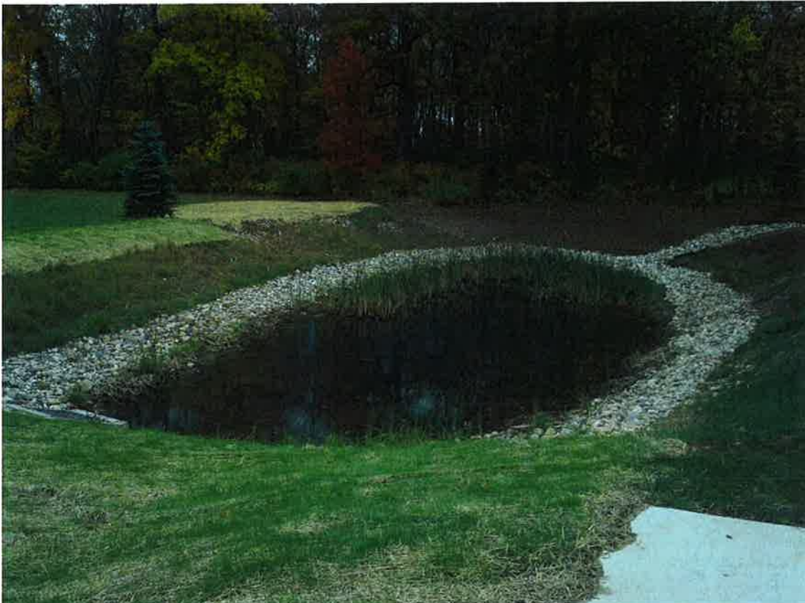
NW of pond, looking south at raised berm with emergency spillway in foreground (Oct. 21, 2013)
