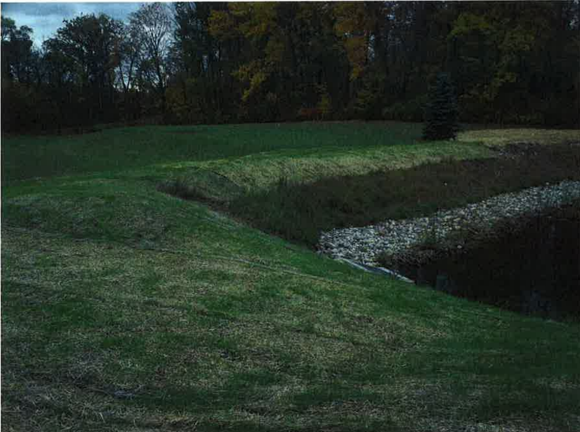
NW of pond, looking east at repaired emergency spillway (Oct. 21, 2013)
