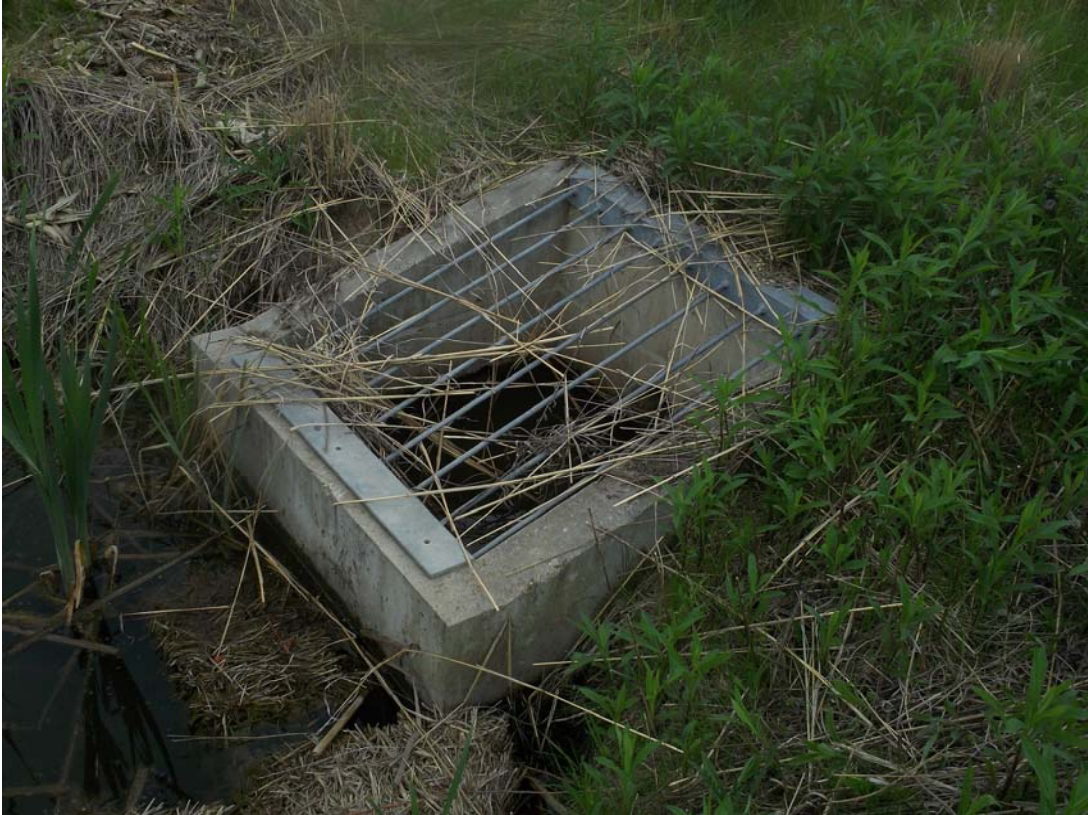
Figure 3: At southeast portion of pond; looking northerly (pond outlet structure)
