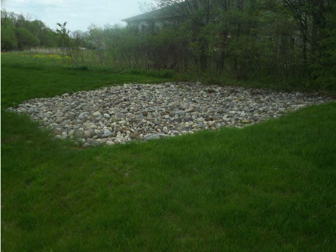
Figure 4: At southeast portion of pond; looking southeasterly (emergency spillway)
