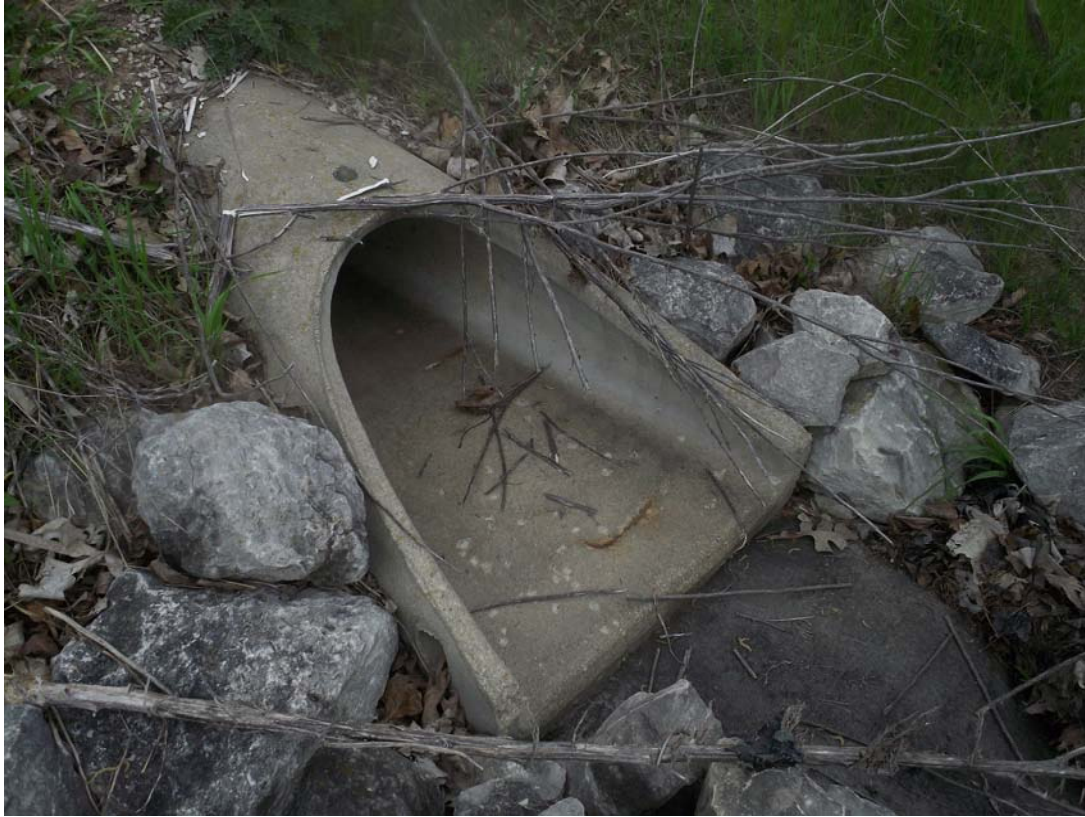
Figure 5: At north portion of pond; looking northwesterly (storm outfall)
