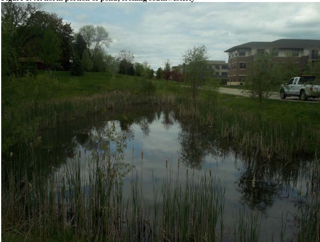
Figure 2: At south portion of pond; looking northerly (two storm outfalls)
