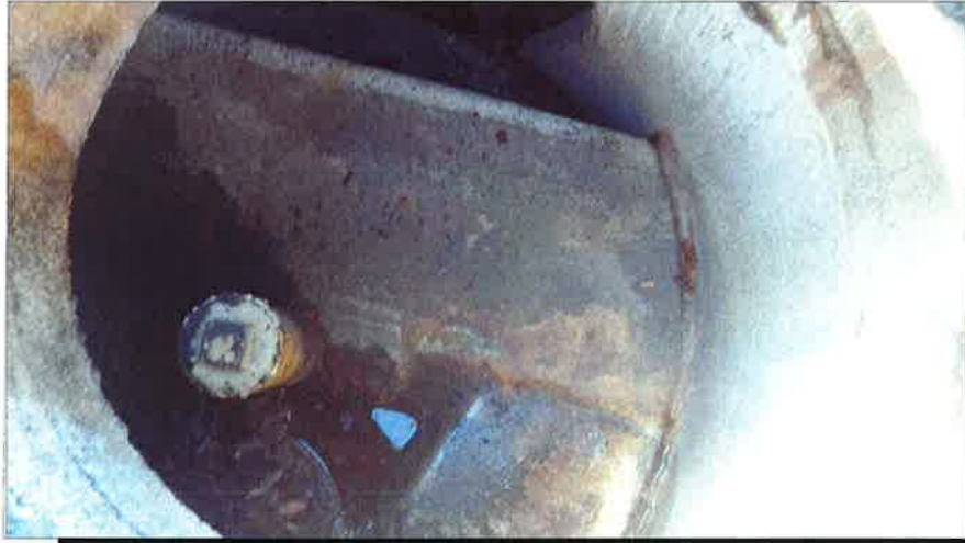
Site Photo 1: April 25, 2014 Stormceptor
