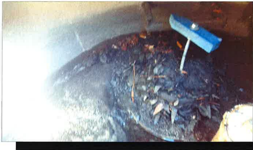
Site Photo 2: April 25, 2014 Stormceptor
