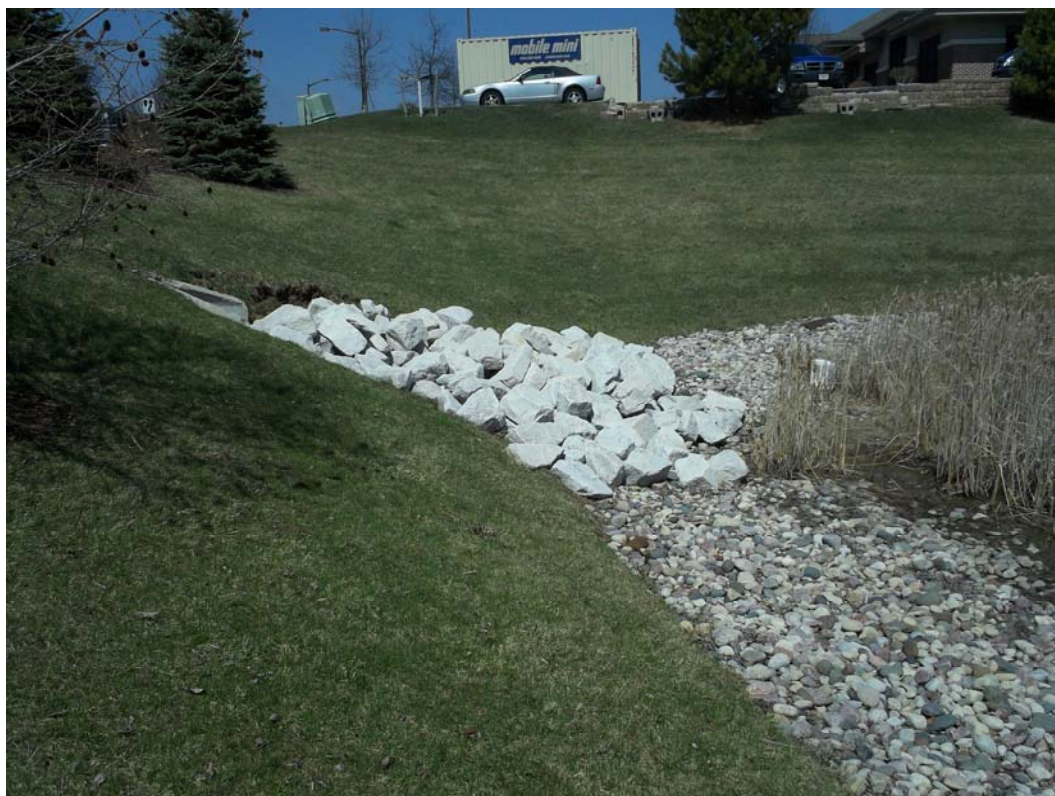
At southwest of pond; looking northerly to storm outfall (rip rap) into pond
