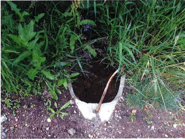
Photo #5: Outfall structure with clear storm water discharge.
