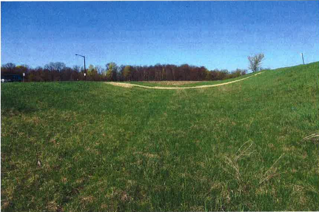
Erosion Control Sediment Trap - Looking west from near outlet pipe.
