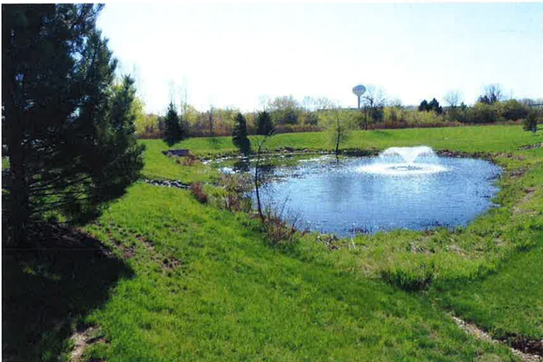
Wet detention pond for Thunder Ridge Drive and Home Depot.
