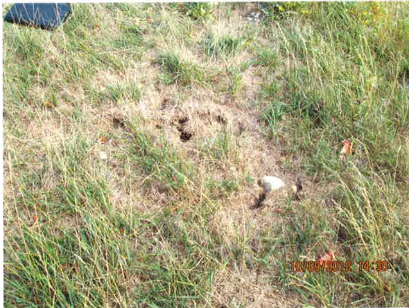
Pond I.D. #SWPO2S002 Localized erosion north side of pond
