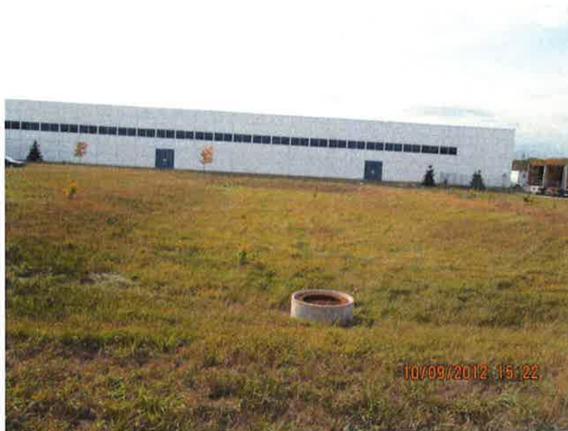
Pond I.D. #SWPO2S001 Looking west across dry basin
