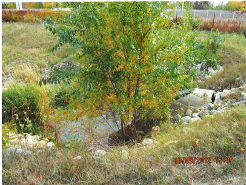
Pond I.D. #SWPO2S002 Woody vegetation by 72-inch outfall into pond
