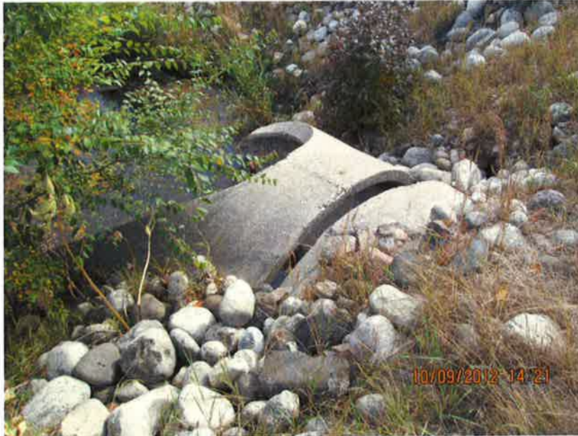
Pond I.D. #SWPO2S002 Disconnected 72-inch outfall to pond
