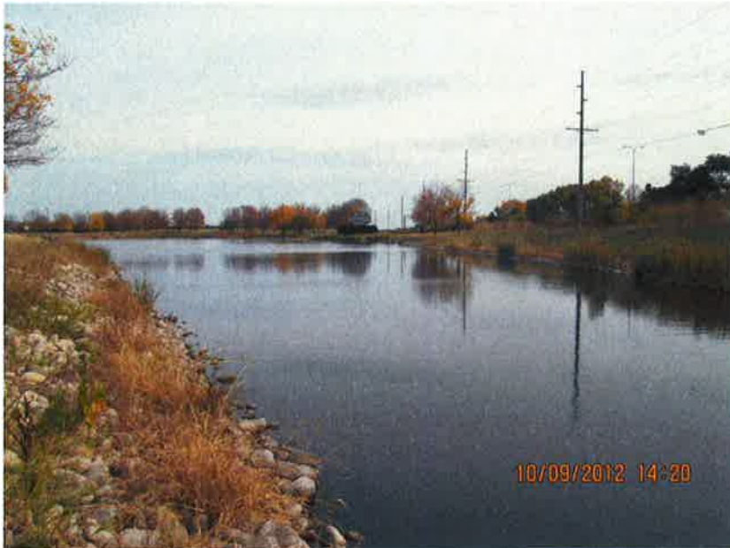
Pond I.D. #SWPO2S002 Looking east across pond
