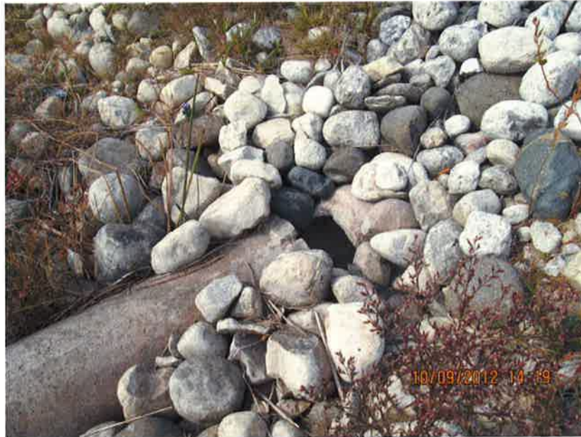
Pond I.D. #SWPO2S002 Disconnected 12-inch outfall to pond
