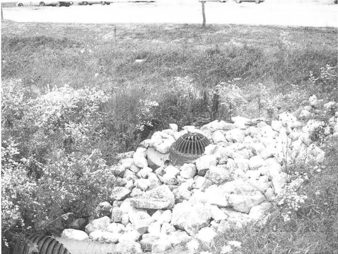
Looking at outlet structure rim from eastern slope
