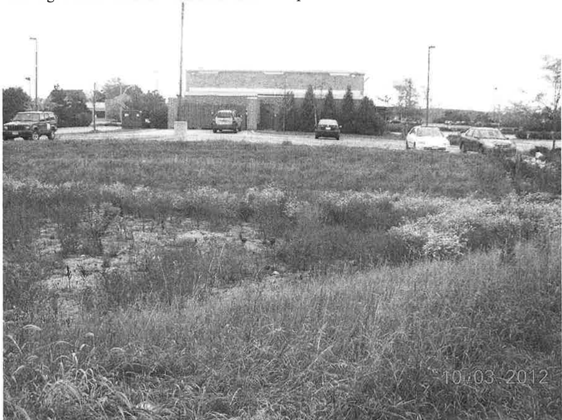
Looking at facility from north slope
