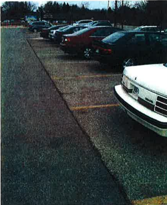
Photo #12: Porous Pavement – looking east at south parking area in front of Building A where the pavement was replaced due to material defects. (good condition)
