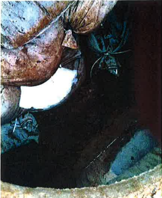
Photo #5: South chamber of outfall structure (sand bags in good condition)
