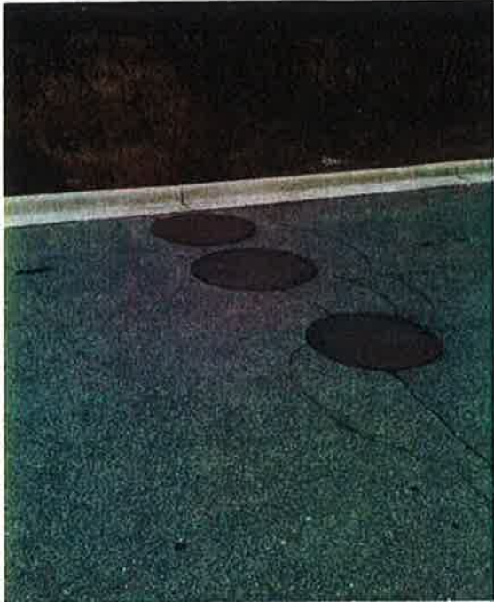
Photo #3: Outfall Structure Manhole Lids
