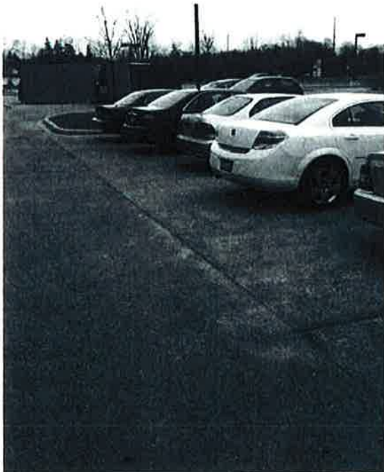
Photo #8: Porous Pavement – looking east at north side of center parking area (area of pavement replacement - good condition)
