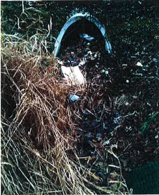
Photo #1: 12" Outfall Structure (looking south and end wall)
