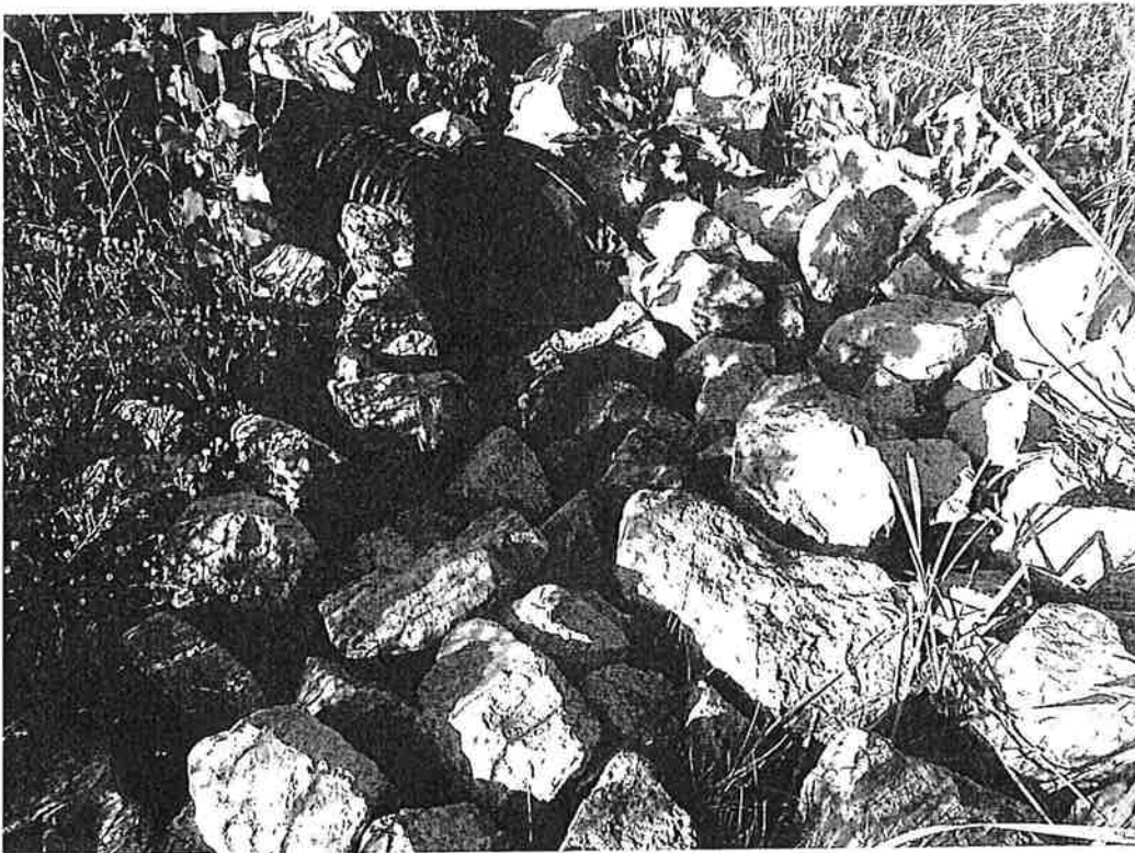
#10 – Temporary sediment basin inlet pipe.
