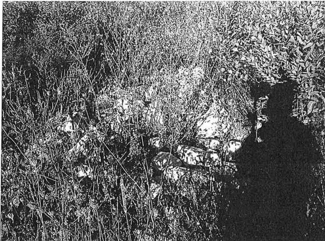
#6 – Emergency spillway, riprap becoming overgrown.
