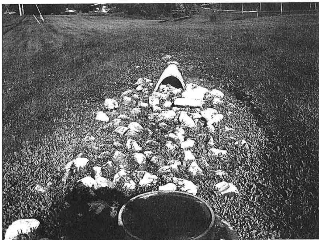
#2 - Downstream end of outfall, riprap getting grown in.
