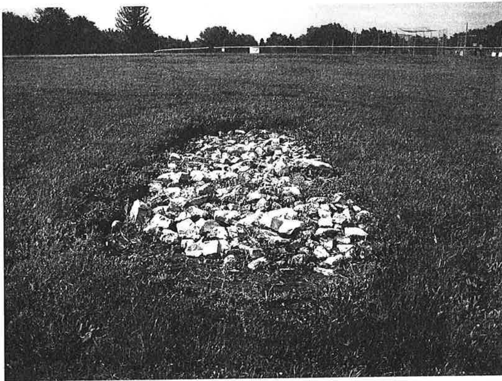
#2 - Storm outfall #1, SE corner of pond, minor areas of dead grass around riprap.
