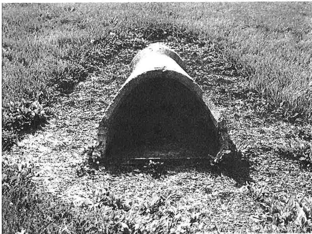
#4 - Upstream end of outfall, Riprap rocks in AEW, grass died around AEW
