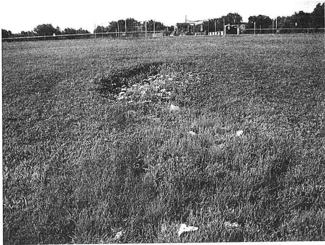
#1 - Storm outfall #2, South side of pond, Minor erosion around riprap, riprap push down slope.
