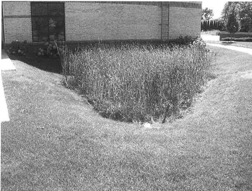
Dry Pond 14N002 looking South
