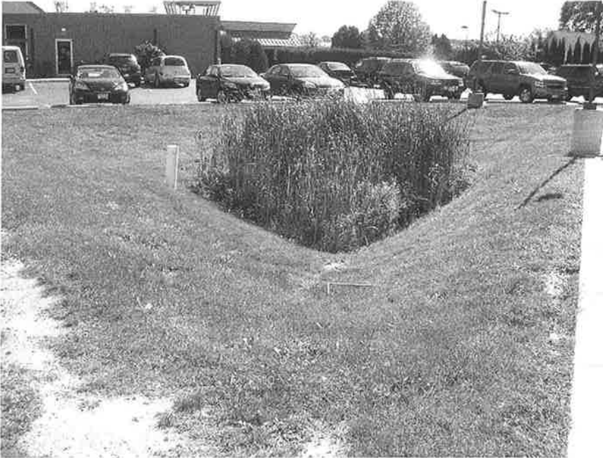
Dry Pond 14N001 looking South
