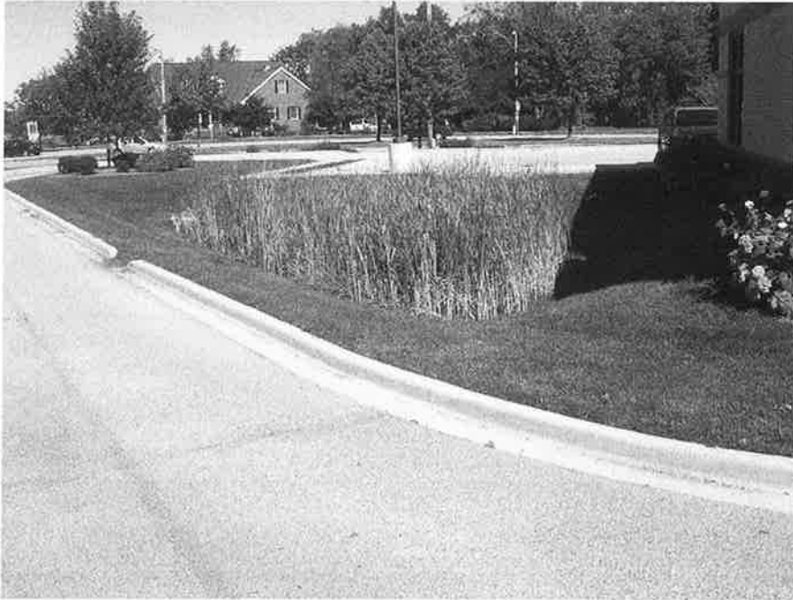
Dry Pond 14N002 looking East
