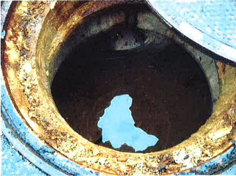
Photo #6: 12" Underdrain collection chamber (good condition)
