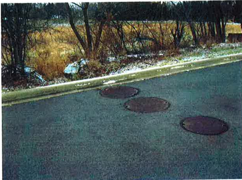
Photo #3: Outfall Structure Manhole Lids
