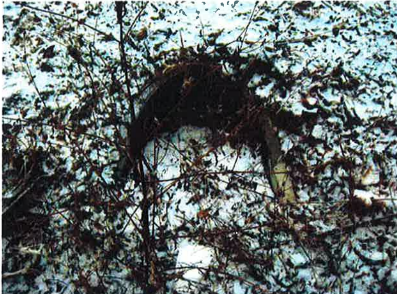
Photo #1: 12" Outfall Structure (looking south and end wall)
