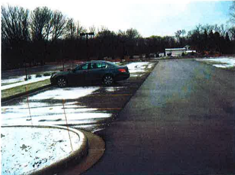
Photo #7: Porous Pavement – looking east at south side of center parking area (good condition)
