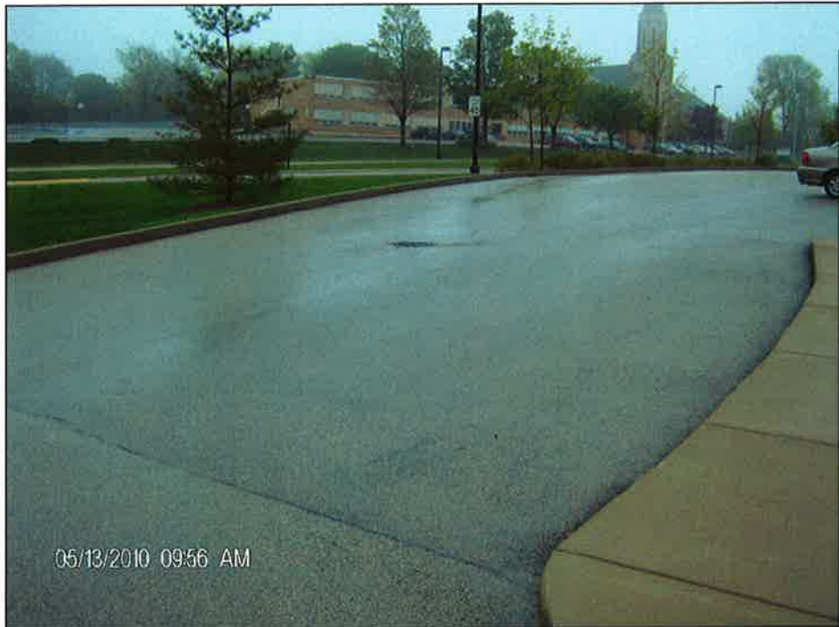
Site Photo 1: May 13, 2010 Stormsewer Inlet
