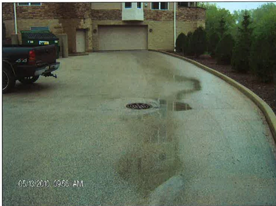
Site Photo 2: May 13, 2010 Stormceptor
