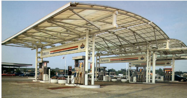
An example of a station that does not have a traditional architectural style, but meets the guidelines. Photo courtesy of Mero Structures, Menomonee Falls, WI.
