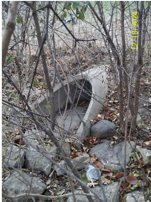
Overflow Outlet ST013448
