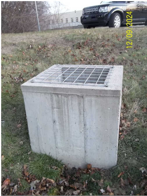
Overflow Structure ST013440
