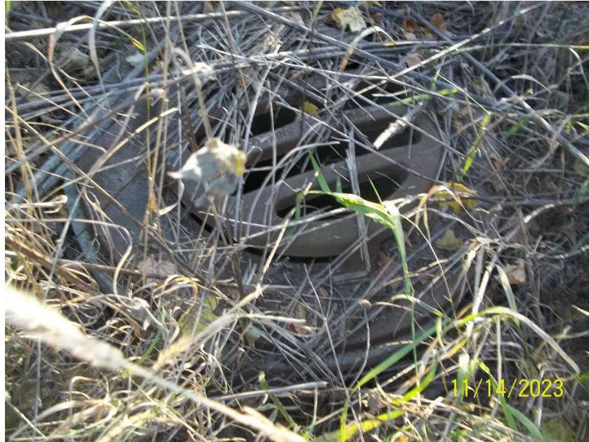
Inlet/Overflow Structure ST015864 to River Outlet
