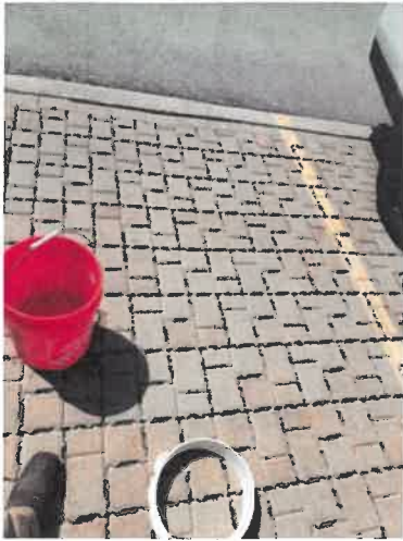
Porous pavement areas drain into existing storm sewer system in Campbell Drive.
