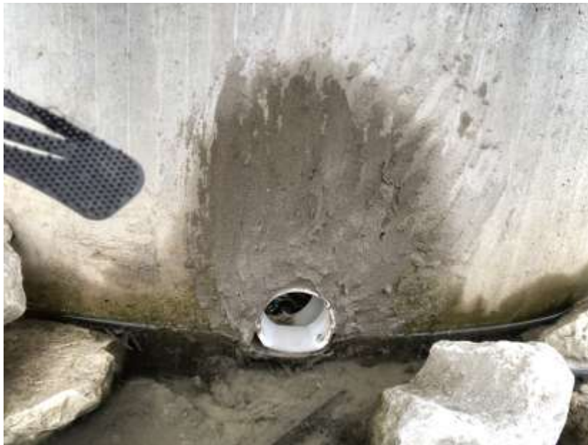
Photo 10: Replaced orifice in NW basin outlet control structure. Photo taken 1/3/20.
