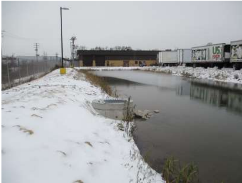
Photo 7: West basin outlet control structure
