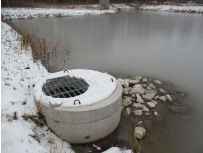
Photo 3: NW storm basin outlet control structure
