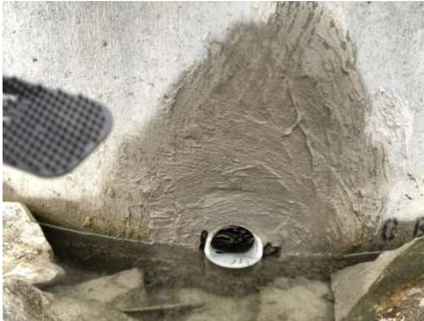
Photo 9: Replaced orifice in west basin outlet control structure. Photo taken 1/3/20.
