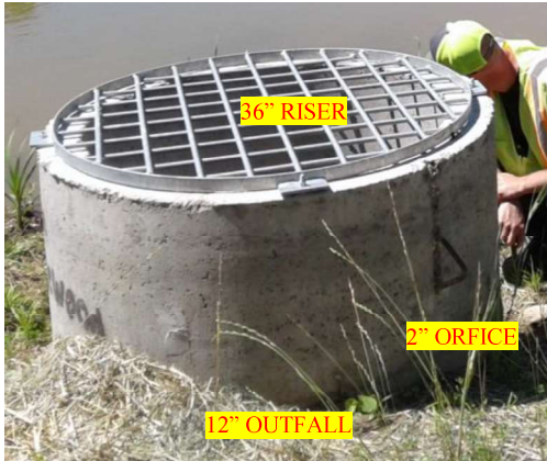
RISER PIPE SIDE VIEW
