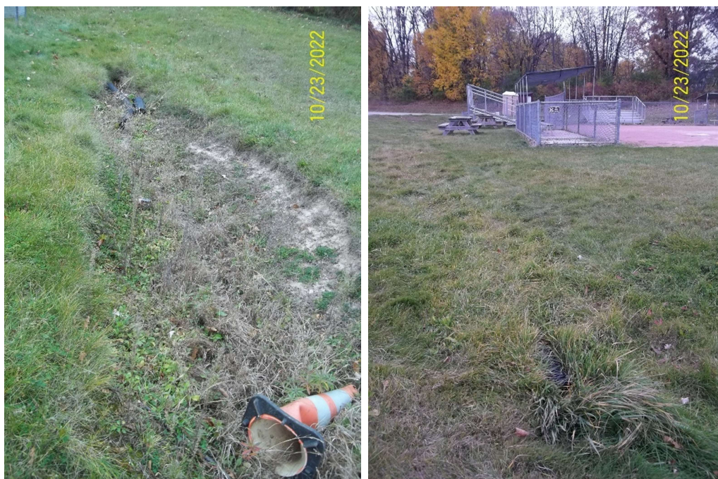
Storm Sewer Outlets ST021162 (North) and ST021163 (South)
