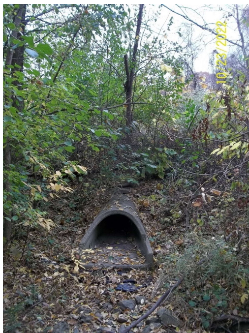
Storm Sewer Outlet ST021160
