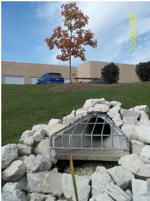
Storm Water Outlet ST015934
