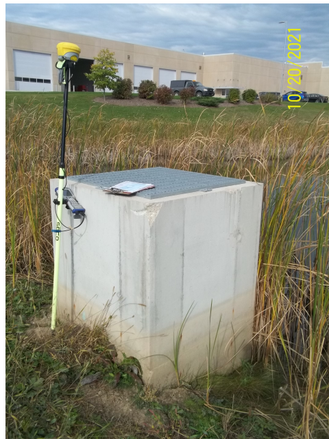
Storm Water Overflow Structure ST014911
