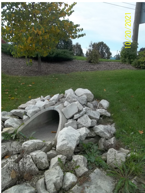
Storm Water Outlet ST015931
