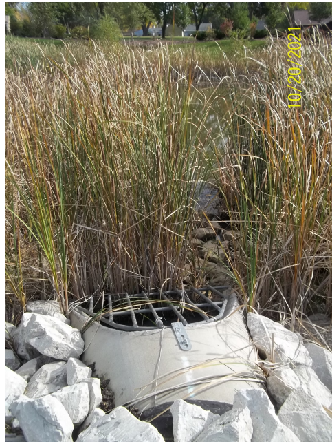
Storm Water Outlet ST015928
