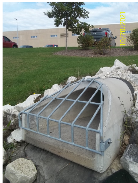
Storm Water Outlet ST015941
