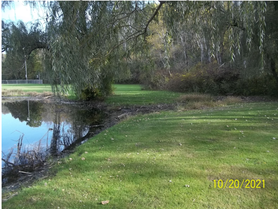
Spillway at E End of Lagoon
